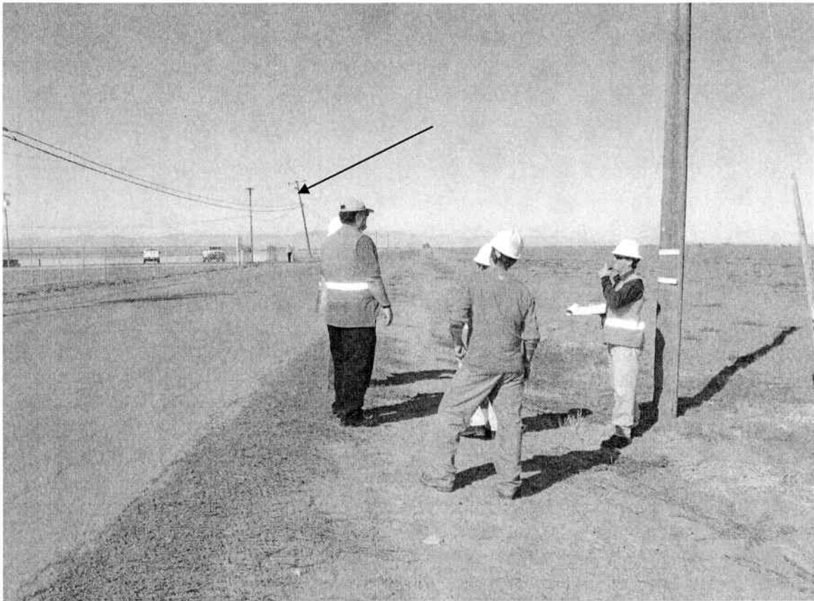
Figure 1 —a leaning pole in Firebaugh.
