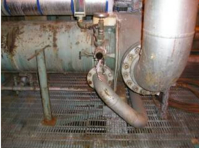
Figure 6. Tape wrapped around exhaust port of Unit 4 steam jet air ejector may indicate prior release of fumes.
