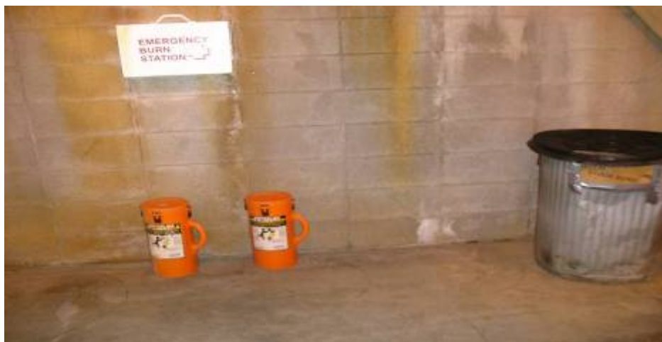
Figure 16. Plant appears orderly and clean.
