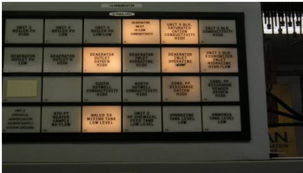
Figure 9. Hydrazine and conductivity alarms activated in the chemical lab.
