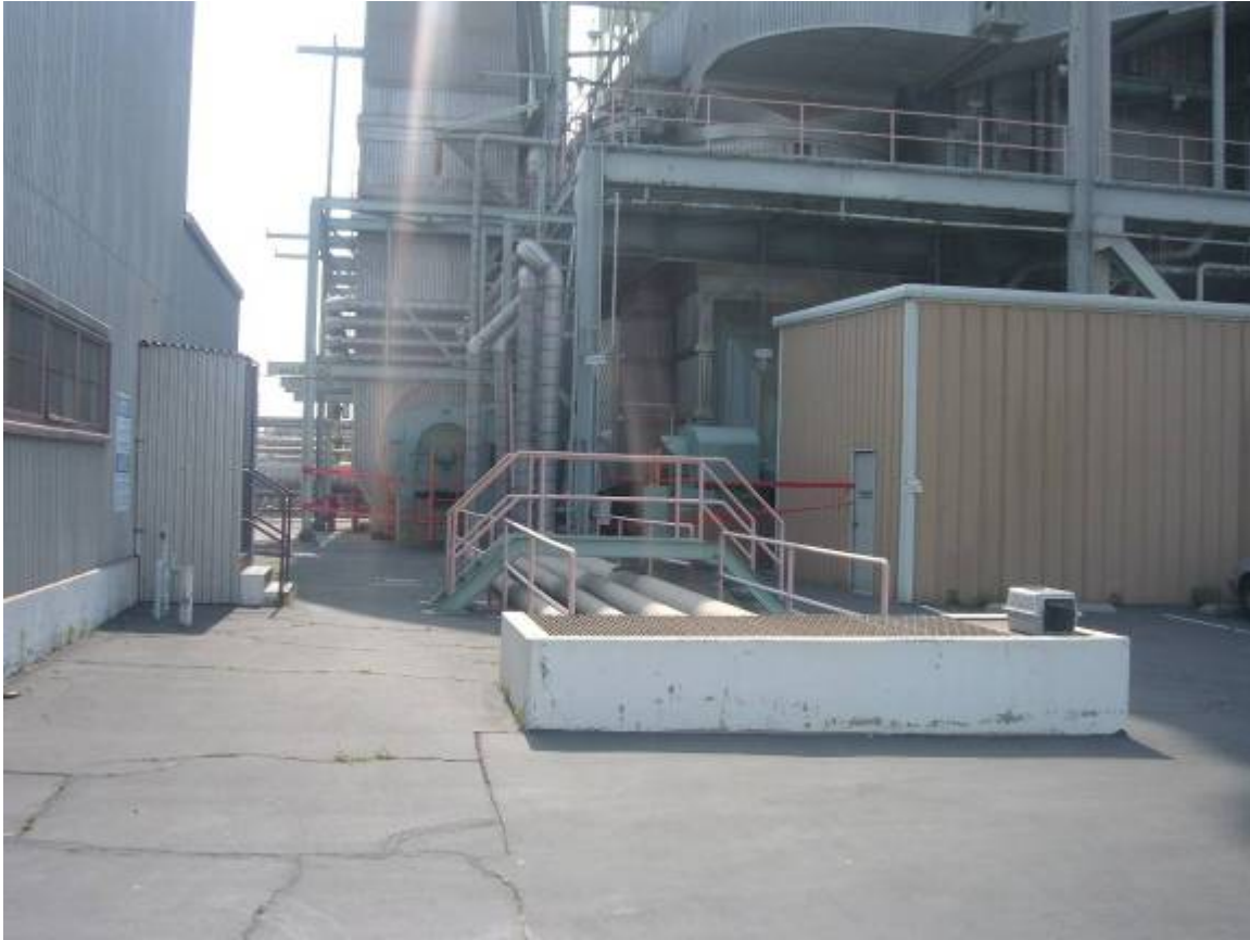
Figure 9. The plant cleaned and placed barricade tape around Units 1 and 2.
