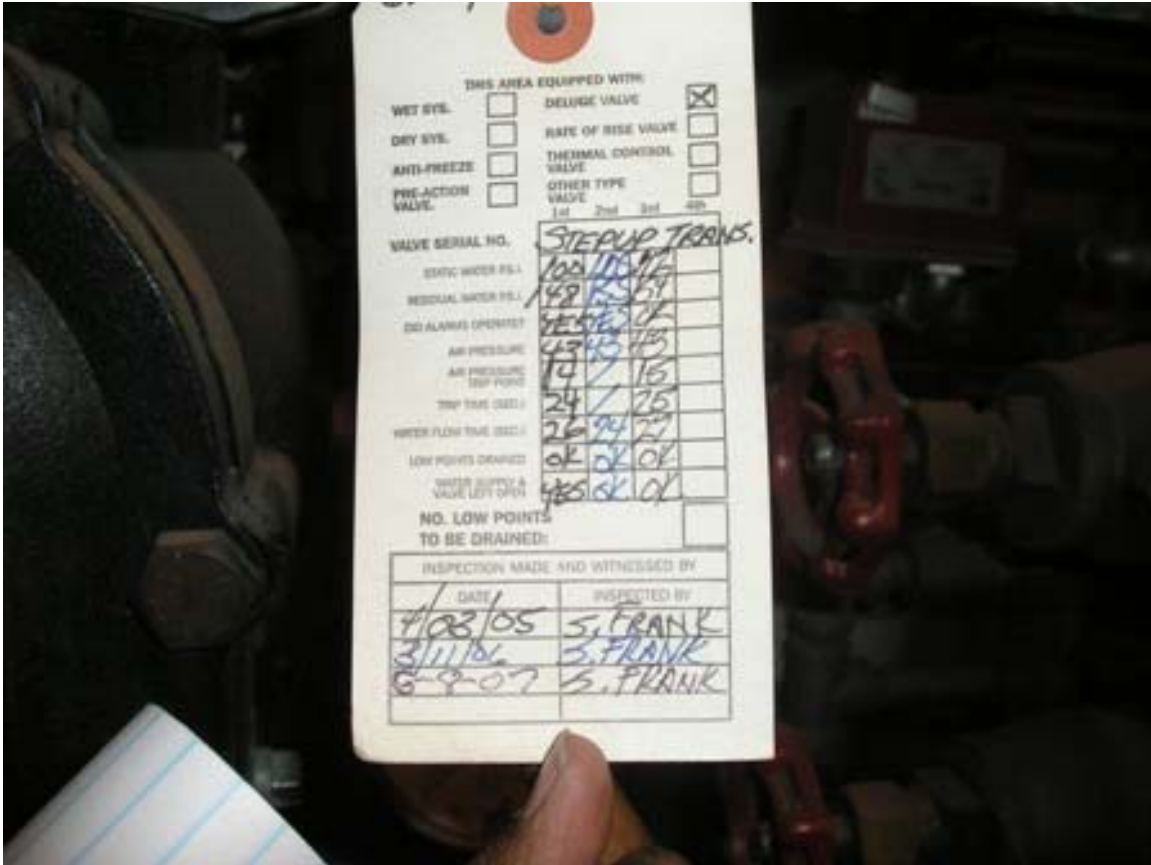
Figure 7. Fire protection systems records show inconsistent dates.
