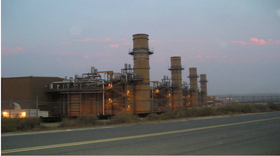
Figure 1. La Paloma Power Plant.
