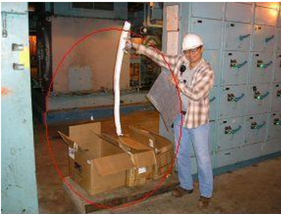
Figure 11. Spill containment dams and absorbent pads are stocked in a highly visible location.
