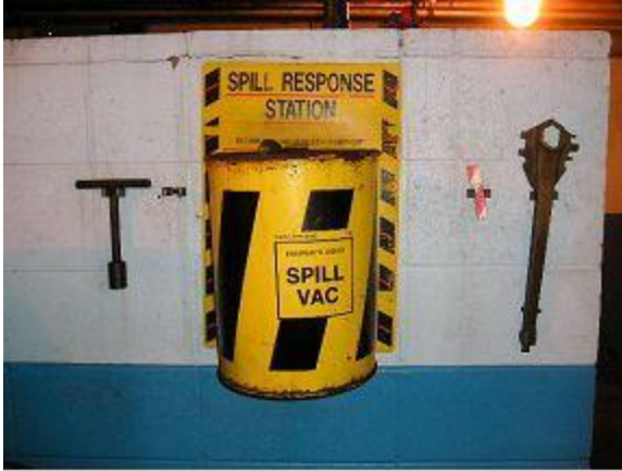
Figure 10: Spill response station is within easy access and is readily available.
