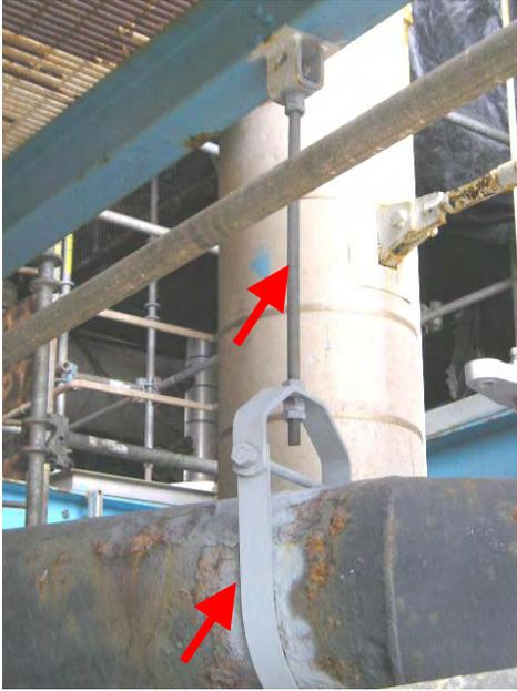
Figure 26 -- This is a photo of a new hanger and pipe support on an older pipe.
