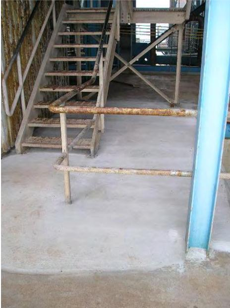
Figure 13 -- The plant was unable to unclog the plugged drain. Rather, the plant applied epoxy cement over it to correct the low spot and allow proper drainage. Also see Figure 9.
