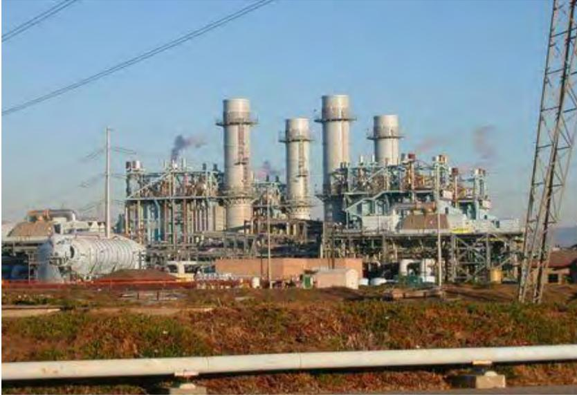
Figure 2 -- Units 1 and 2 are new, combined-cycle units.
