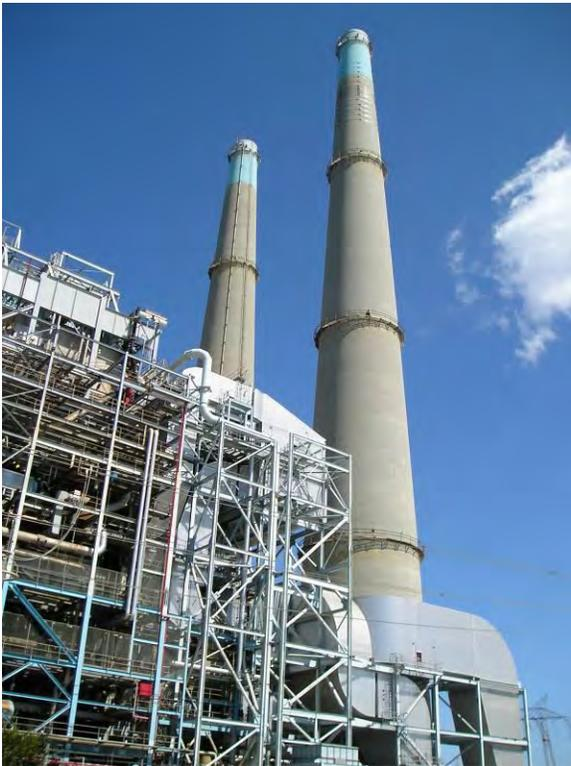
Figure 3 -- Units 6 and 7; conventional, once-through, supercritical boiler units.
