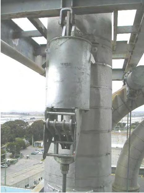
Figure 22 -- Close-up view of a new spring support.
