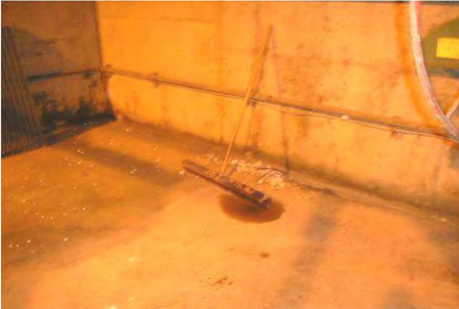
Figure 11 -- Insulation from the over head pipe; no asbestos containment precautions are evident.
