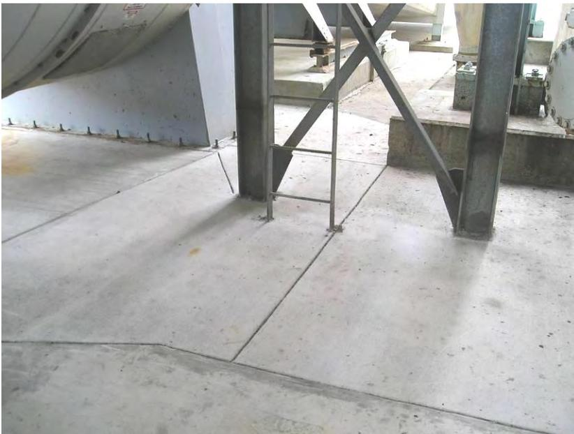
Figure 14 -- To prevent water accumulation, the plant used epoxy cement to re-grade the area for proper drainage.
