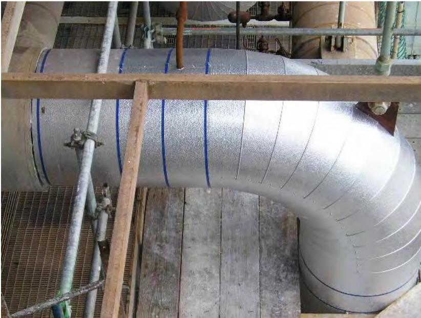
Figure 16 -- Plant staff used blue banding and dimpled aluminum wrapping to indicate non-asbestos pipe insulation.
