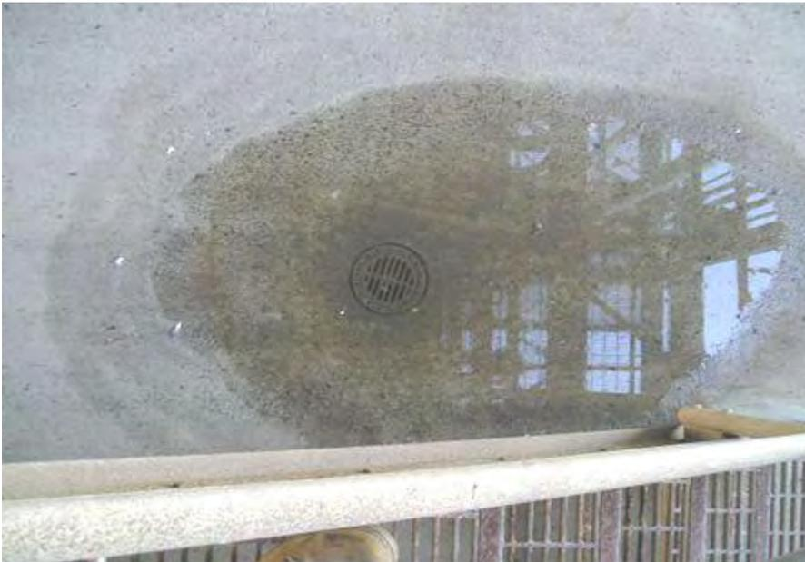
Figure 9 -- Standing water caused by a clogged drain on Level 88 of Units 6 and 7.
