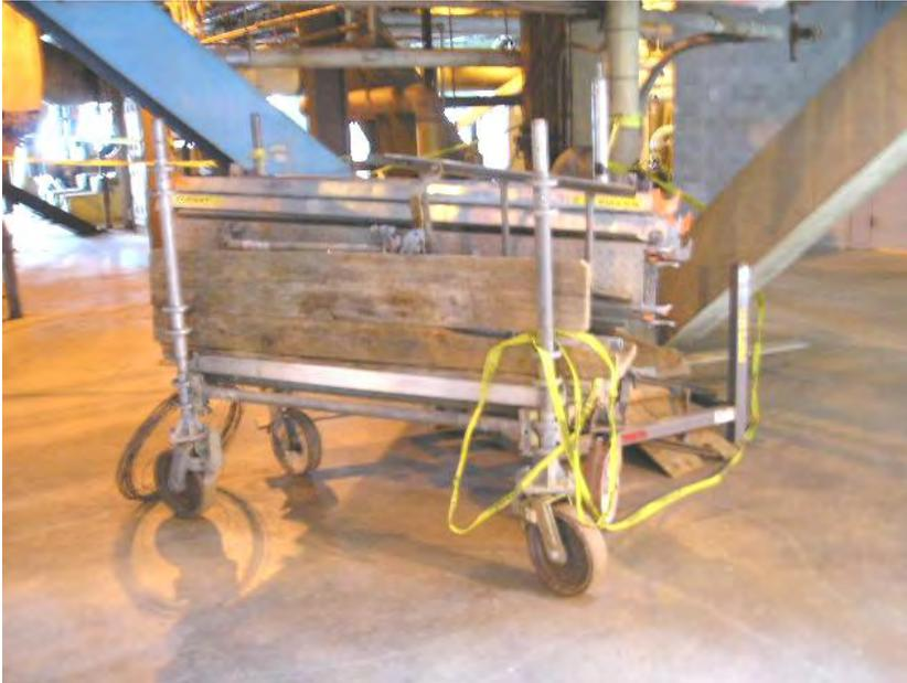
Figure 12 -- Scaffolding carts could be seen in many areas. These carts are surrounded with caution tape when the scaffolding is not in use. The yellow caution tape can be seen in this photo.
