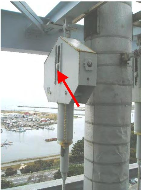
Figure 23 -- This is a close-up view of a simple spring support with the load indicator in the center of the polygon.
