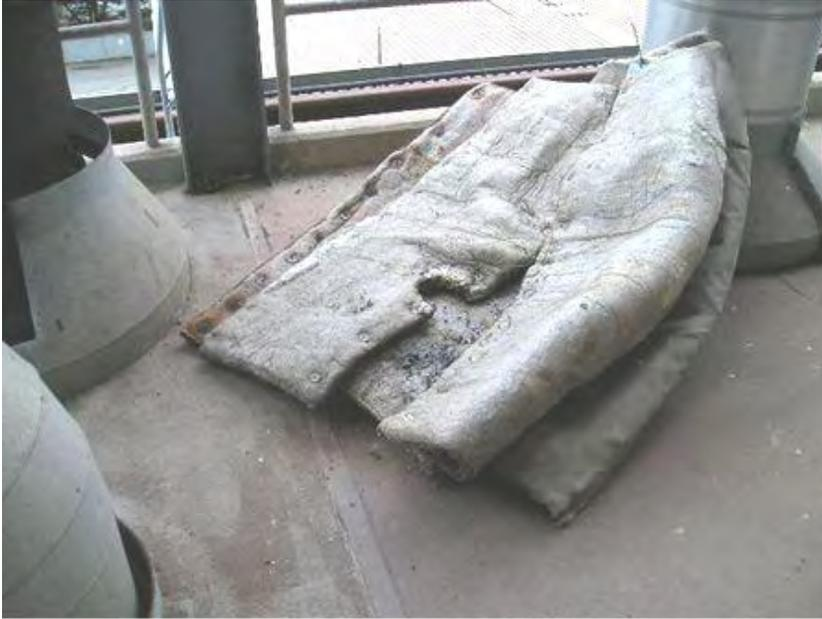
Figure 8 -- Insulation, possibly containing asbestos, on Level 104 of Units 6 and 7.
