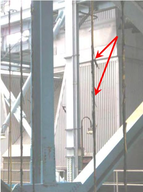
Figure 20 -- Severely deteriorated pipe hanger rods visible from Level 102 of Units 6 and 7.
