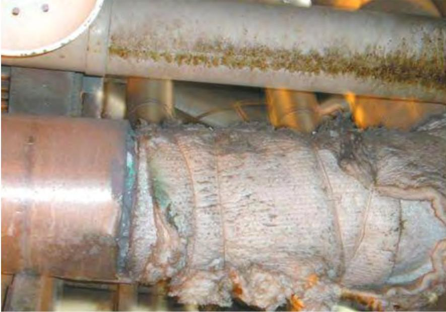
Figure 10 -- Frangible insulation falling off an exposed pipe in the basement of Units 6 and 7. The pipes lack blue banding, which would indicate the absence of asbestos. Therefore, asbestos is assumed to be present.
