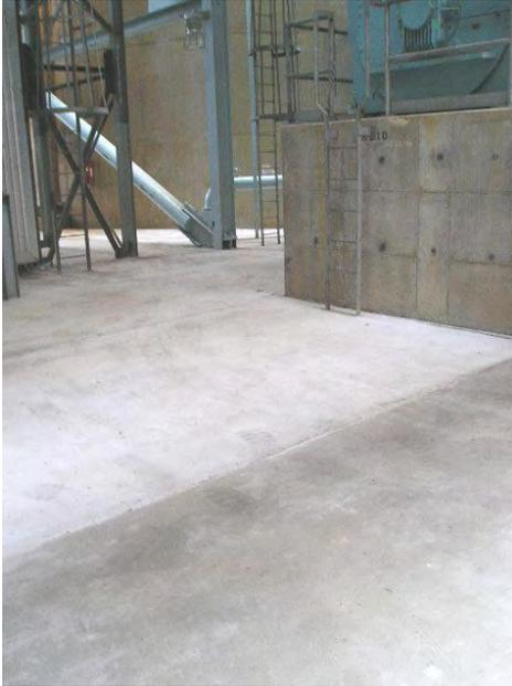
Figure 15 -- To prevent water accumulation, the plant used epoxy cement to re-grade the area for proper drainage.
