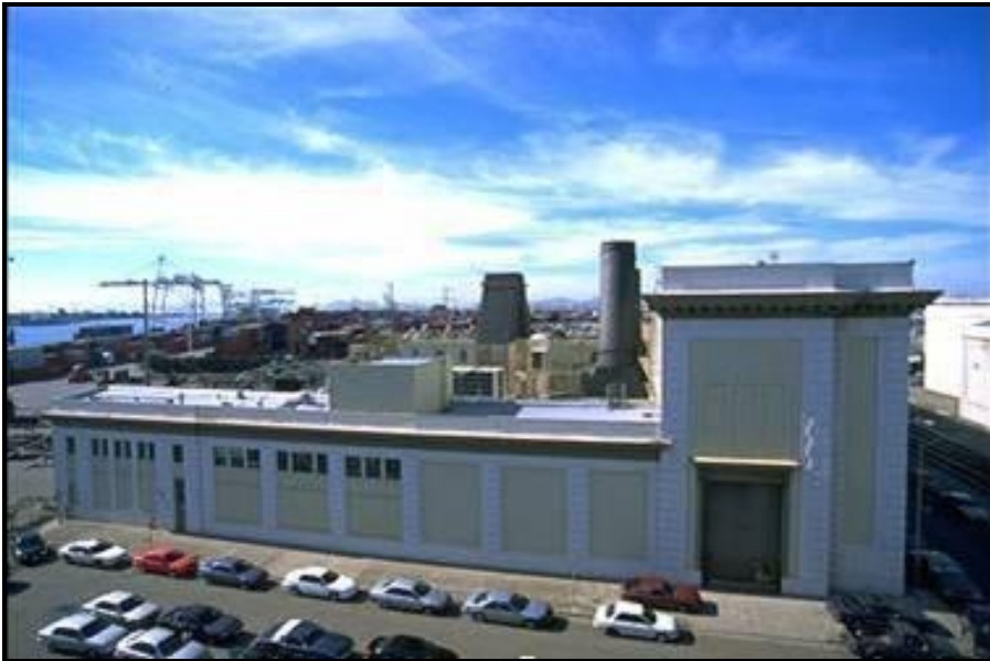
Figure 1 -- Oakland Power Plant as seen from atop an oil storage tank. Photo: LS Power Group ( http://www.lspower.com/projects/ )
