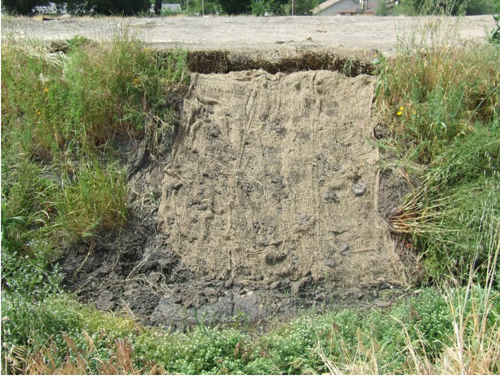
Figure 1 – Repaired bank of Drainage #30, May 12, 2006.
