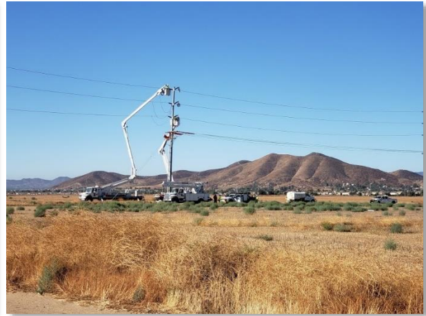
Figure 6. Reconducting activities from Construction Area UNK250 to UNK01
