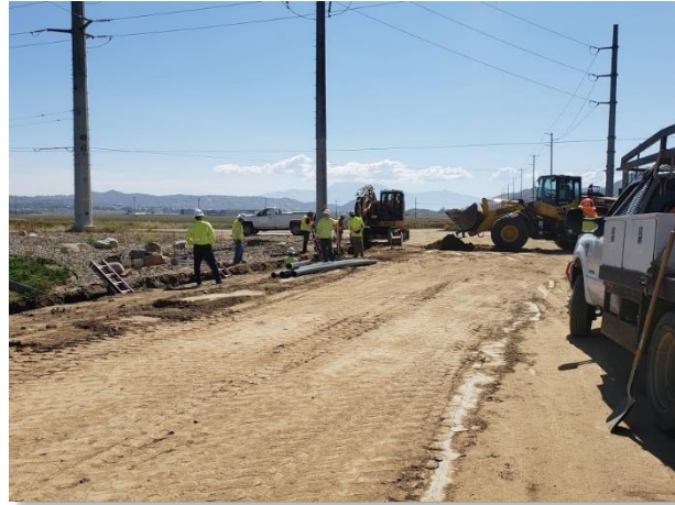
Figure 9. Underground trenching from Valley Substation to Menifee Road
