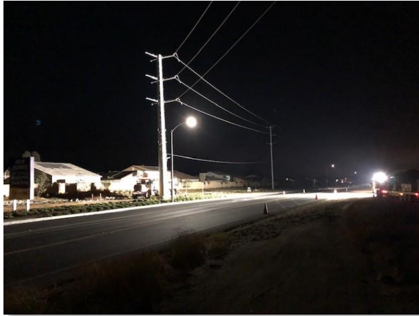
Figure 12. Construction night lighting directed at residences during overnight construction activities from Construction Areas UNK250 to UNK01
