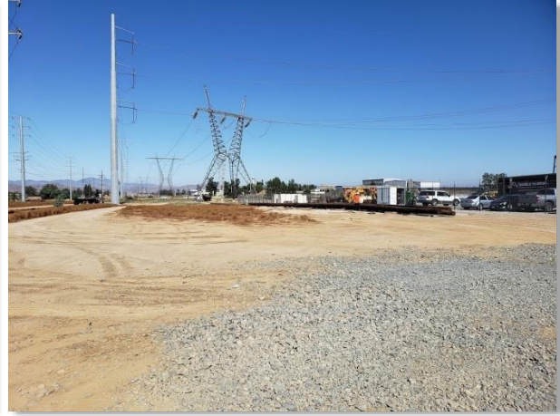
Figure 4. MPC #2 laydown area for wood pole storage
