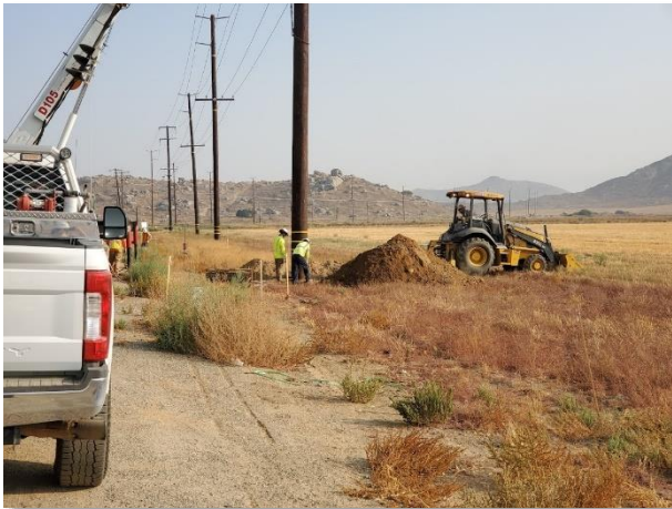
Figure 7. Pole realignment at Construction Area UNK101
