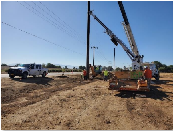
Figure 5. Setting wood pole at Construction Area UNK183
