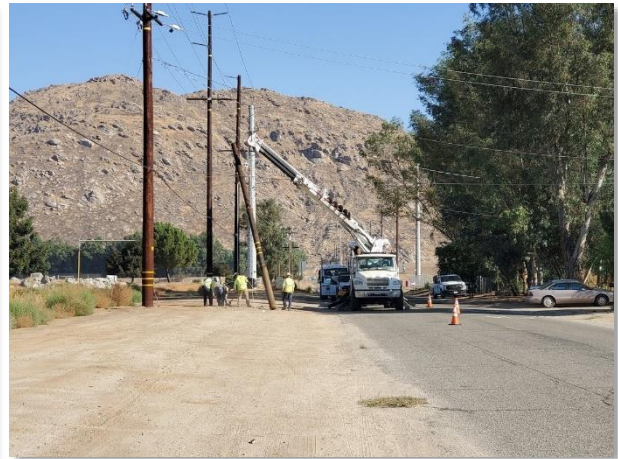
Figure 8. Pole butt removal at Construction Area UNK21
