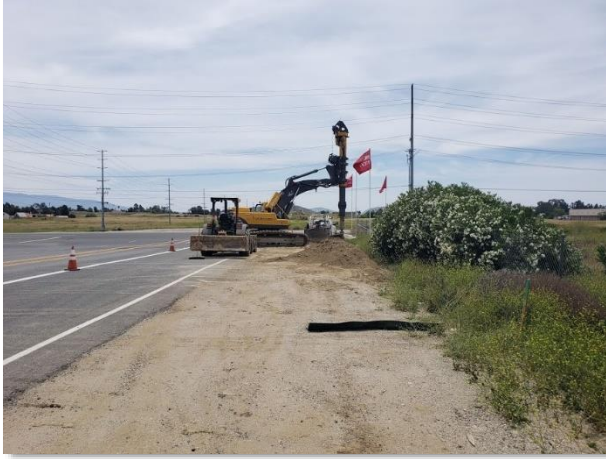
Figure 3. Foundation drilling at Construction Area UNK247
