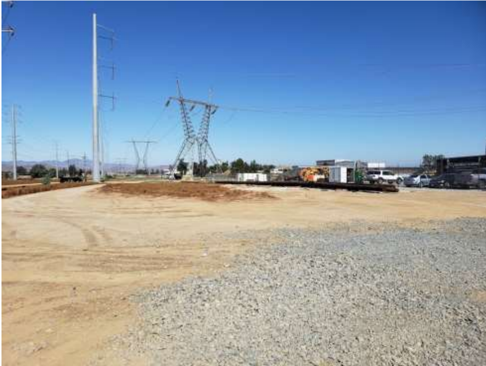
Photo 1 – MPC #2 laydown area for wood pole storage (June 17, 2019).
