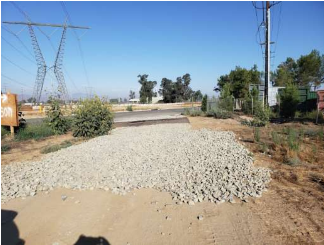
Photo 3 – Valley Yard construction entrance with SWPPP TC-1 required stabilization (July 31, 2019).
