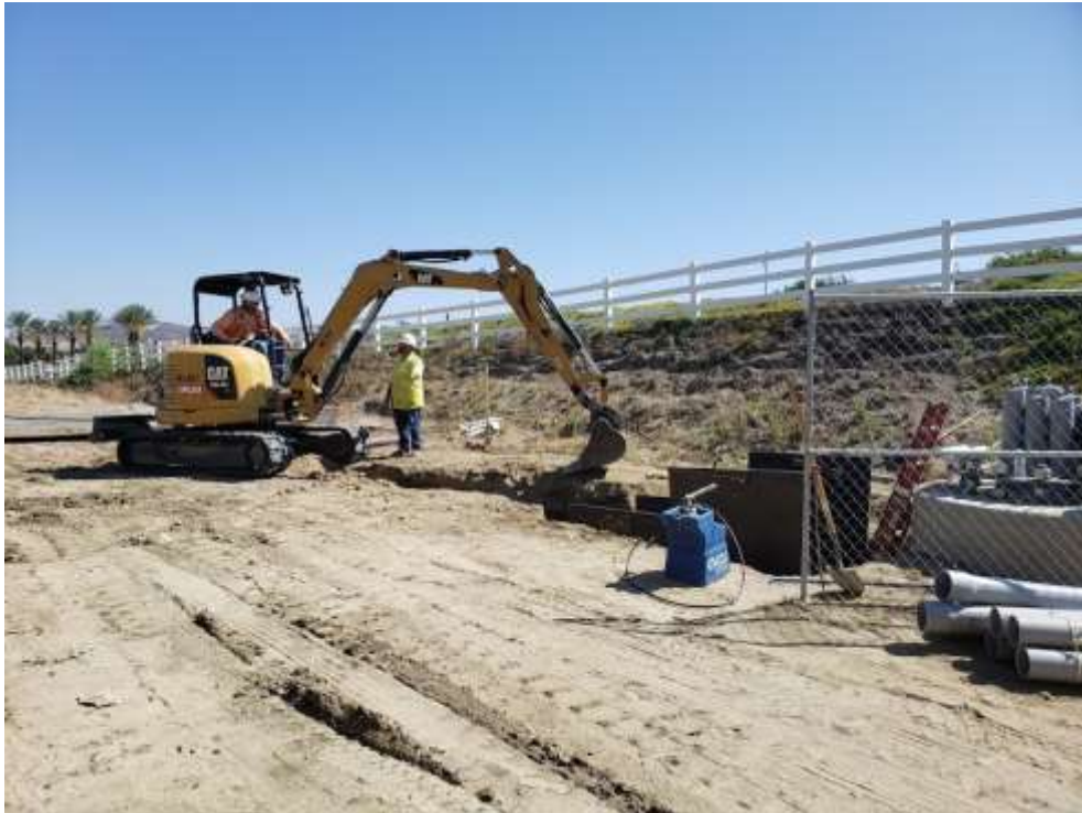
Photo 1 – Trenching from Vault 3 to UNK222 (August 28, 2019).
