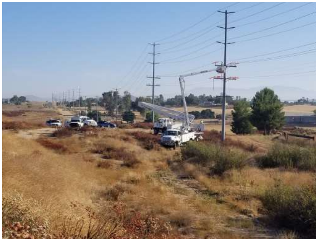
Photo 4 – Lowering crossarms on Segment 2 (Photo courtesy of SCE).
