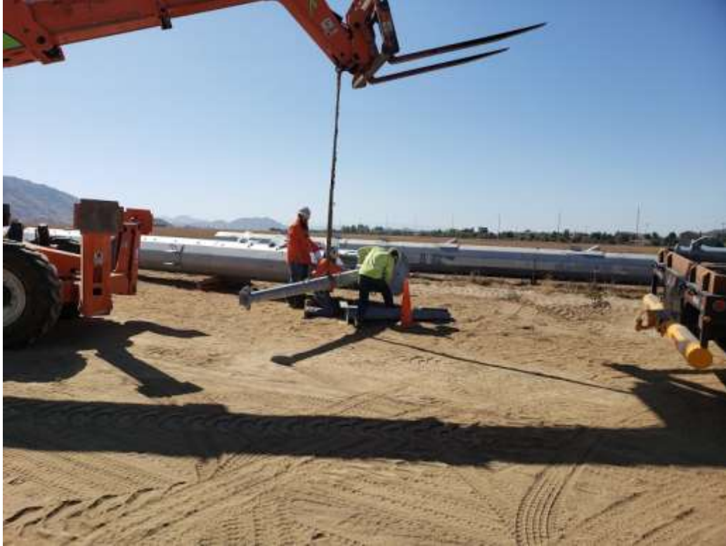
Photo 3 - Framing pole at UNK250 (August 28, 2019).
