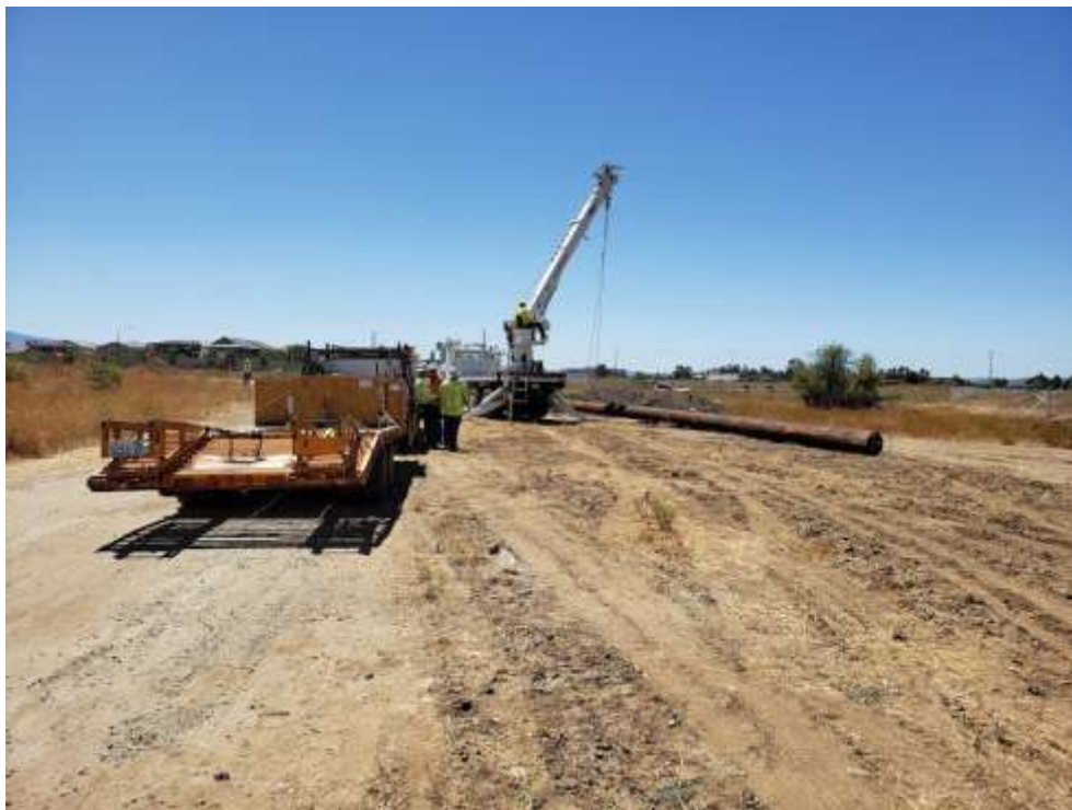
Photo 2 – Setting a wood pole at UNK240 (August 20, 2019).
