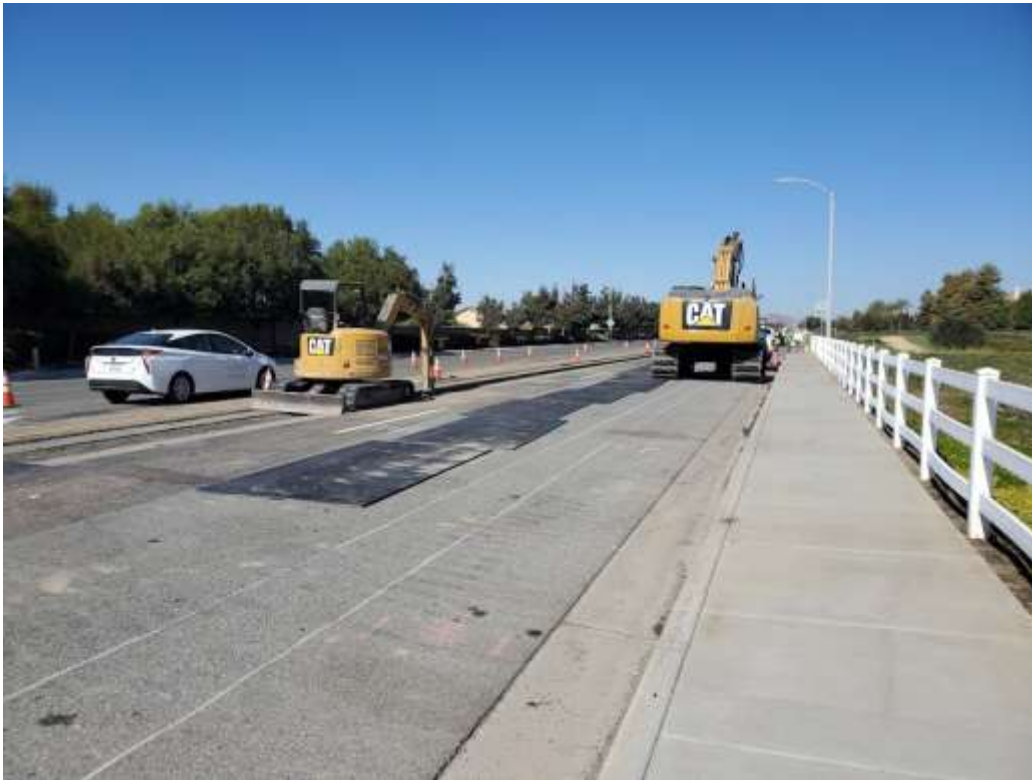
Photo 1 – Construction activities on the southern underground (November 6, 2019).
