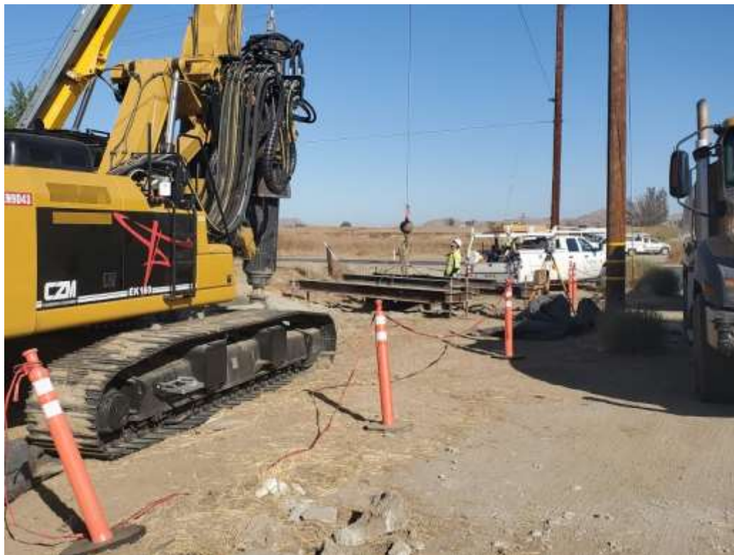
Photo 2 – Foundation activities at Construction Area UNK155 (October 28, 2019).
