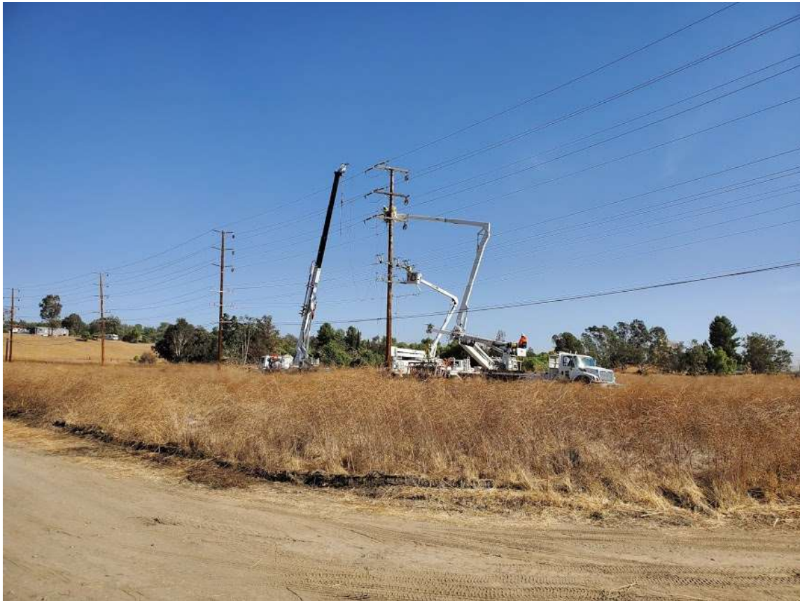
Photo 3 – Reconducting activities on Segment 2 (October 30, 2019).
