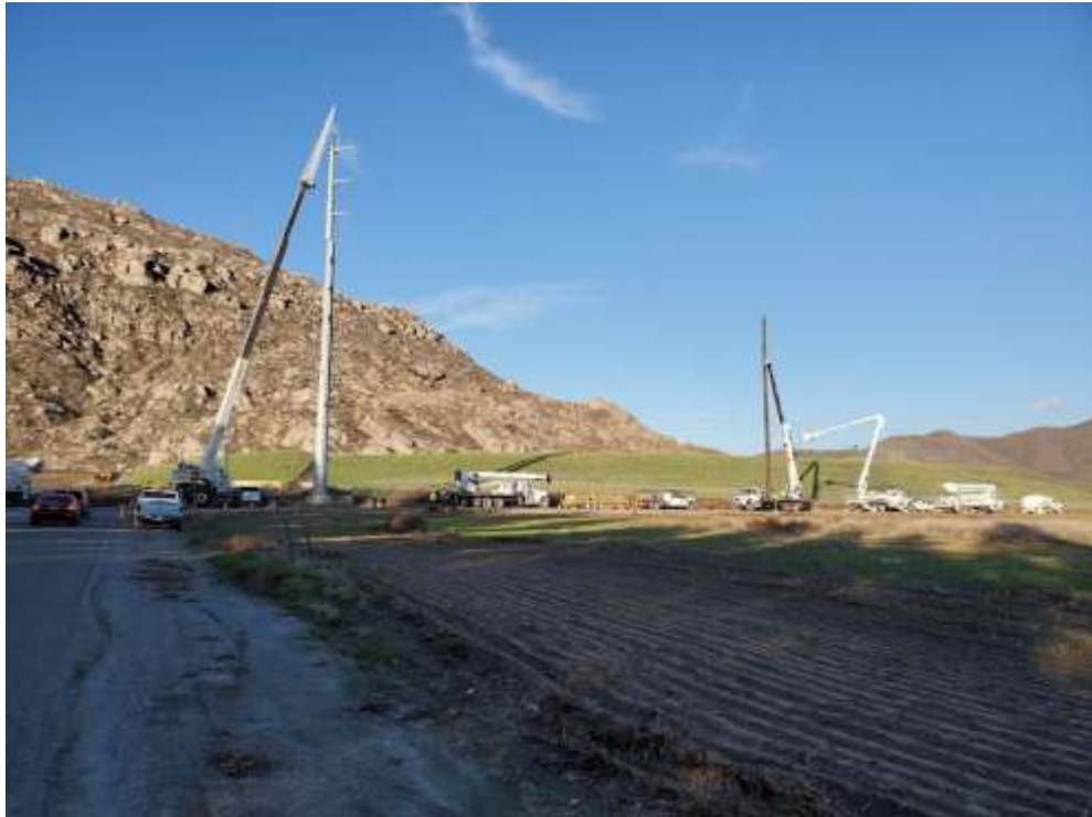
Photo 1 - Assemble of UNK07, and digging and setting pole 1976117E (December 9, 2019)
