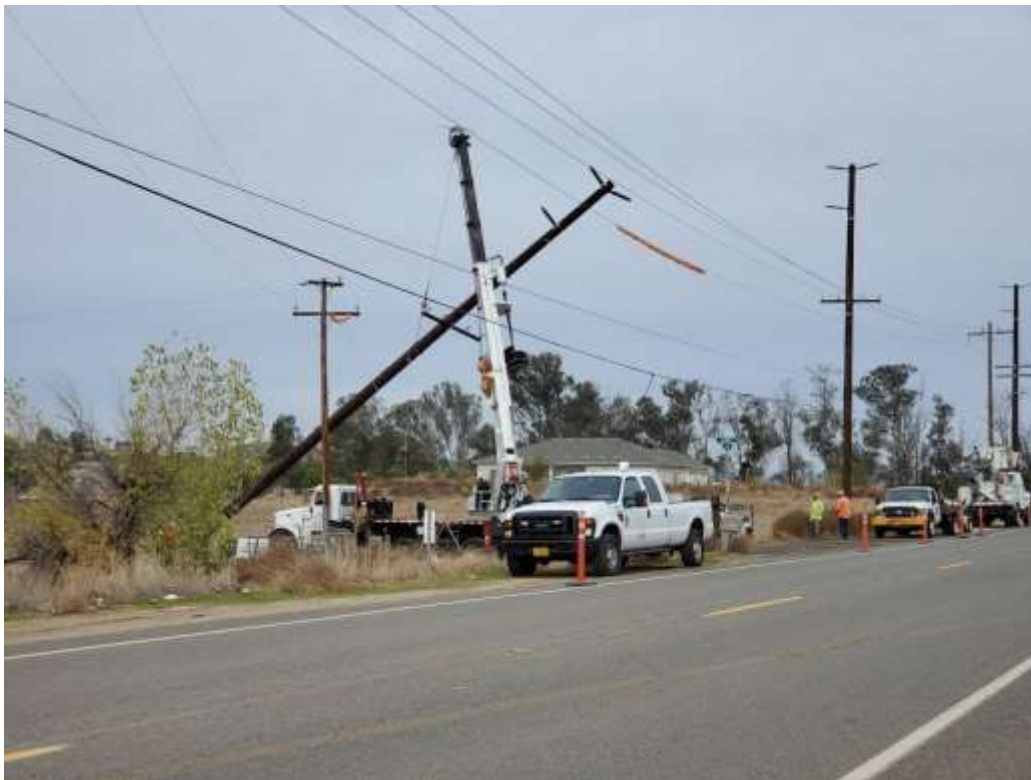
Photo 2 - Digging and setting wood pole (December 3, 2019)
