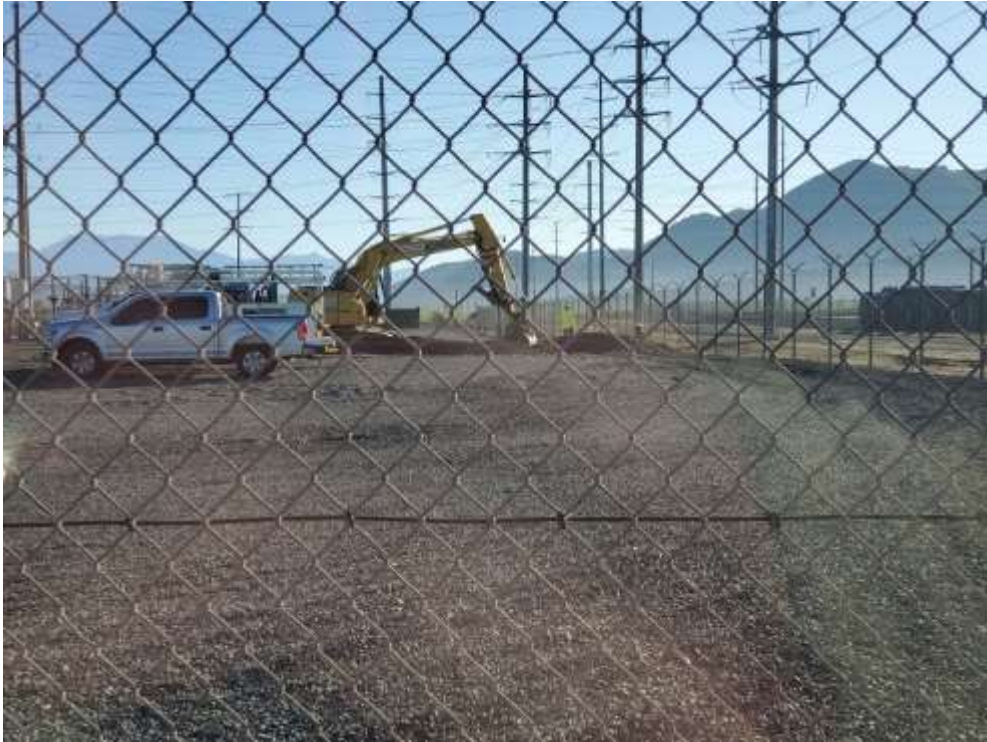
Photo 3 – Trenching within the Valley Substation (January 28, 2020).
