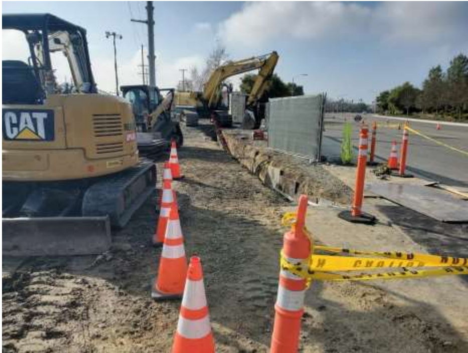
Photo 1 – Trenching and conduit installation on the southern underground (January 22, 2020).
