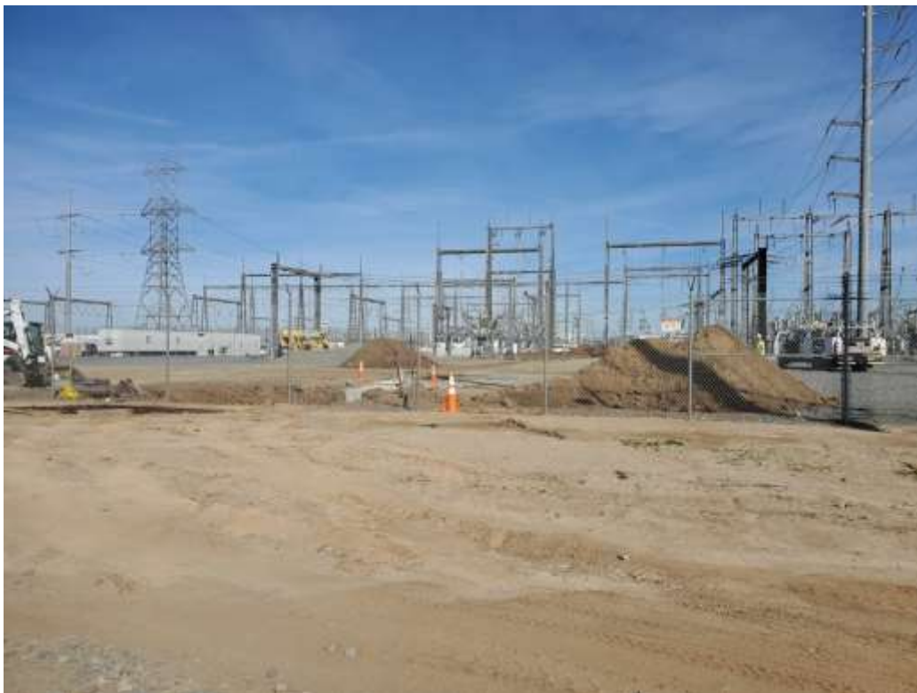
Photo 4 – Trenching and conduit installation within the Valley Substation (February 5, 2020).
