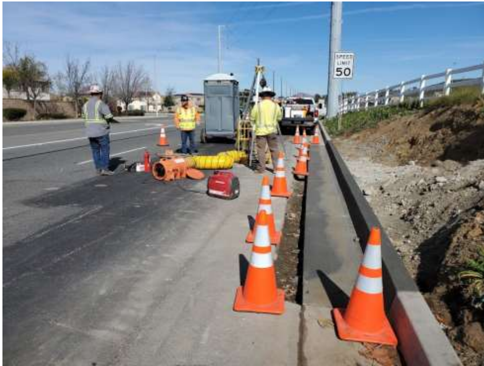
Photo 1 – Vault QA/QC on the southern underground (February 5, 2020).
