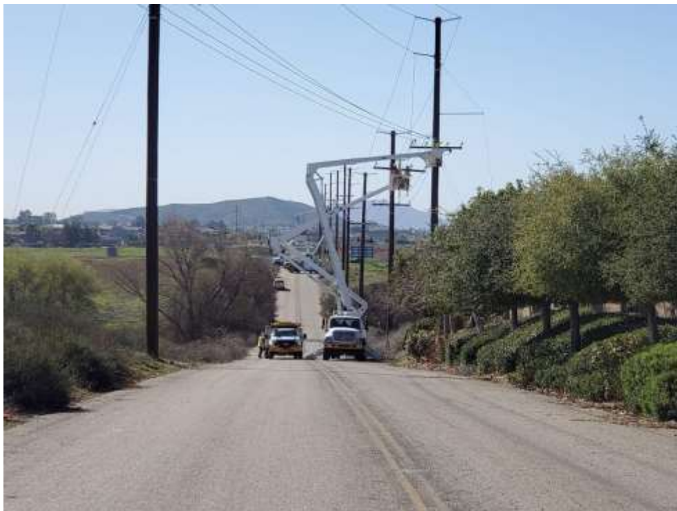
Photo 2 – Distribution wire stringing activities at Construction Areas UNK223 through UNK234 (February 12, 2020).
