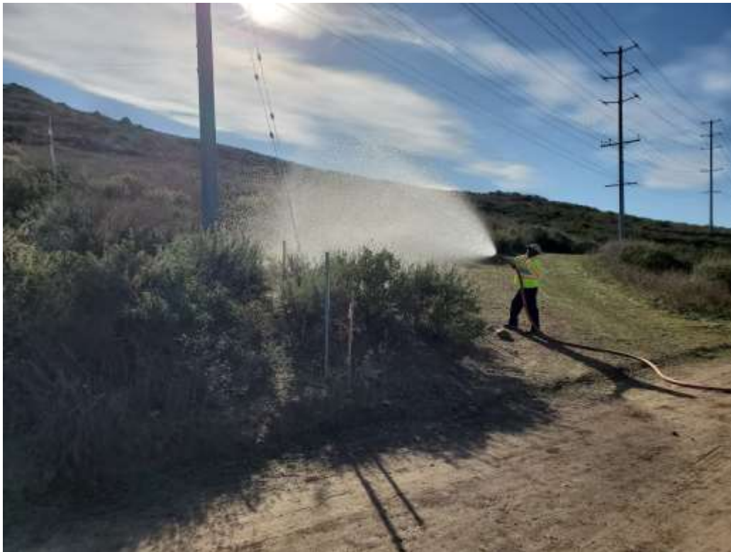
Photo 3 – Hydroseed watering at restoration site (February 12, 2020).
