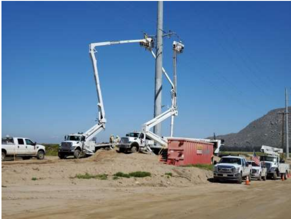
Photo 1 – Wire stringing activities at Construction Area UNK20 through UNK46, Segment 1 (April 1, 2020).
