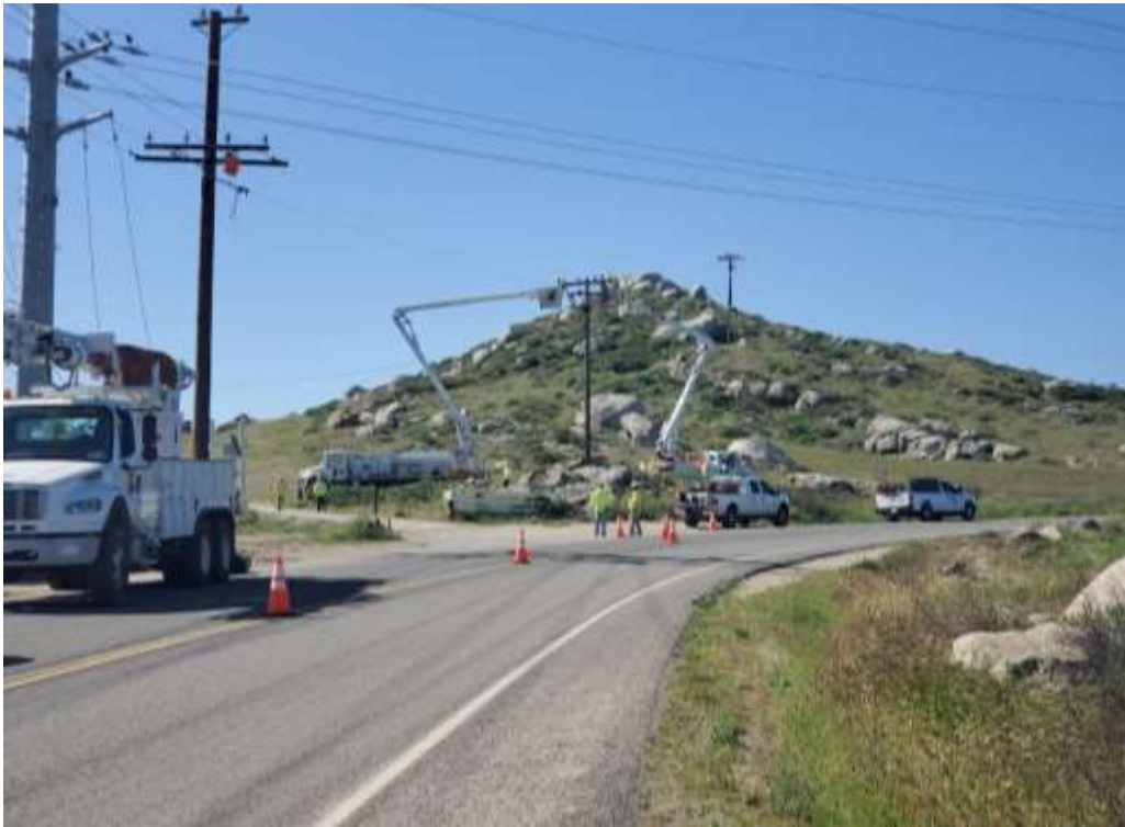
Photo 1 – Reconductoring activities at Construction Area UNK115 to pole 2105782E (April 22, 2020).
