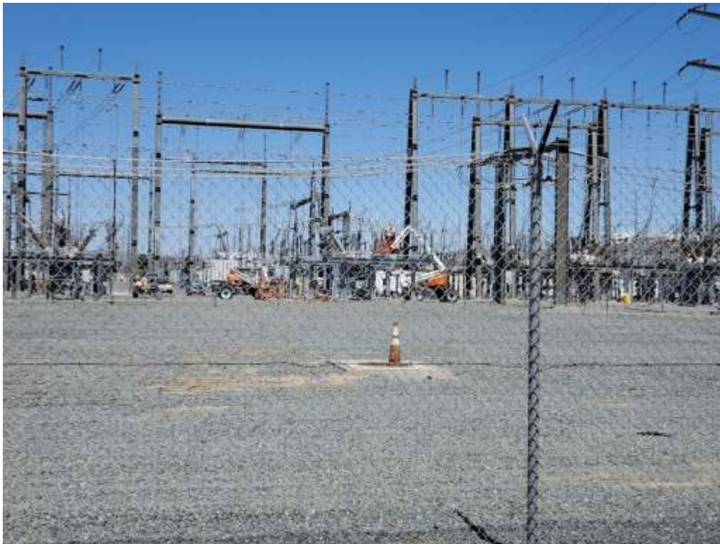
Photo 3 – Construction activities on the 115 kV rack within the Valley Substation (April 15, 2020).
