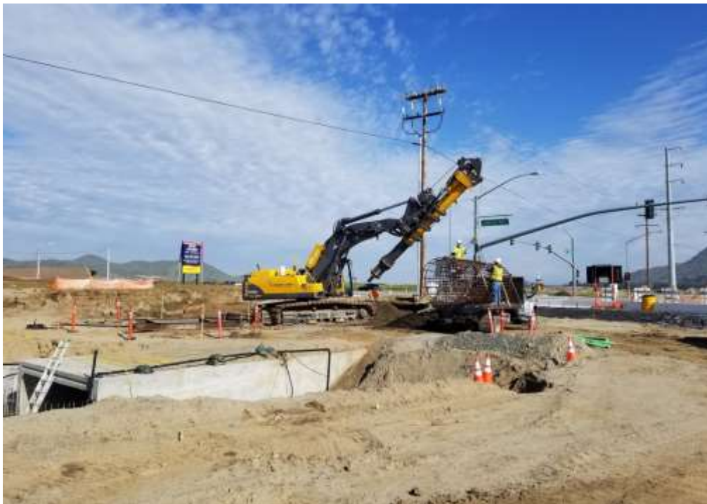
Photo 2 – KV Structures foundation activities at UNK47 (April 17, 2020) (Photo courtesy of SCE).
