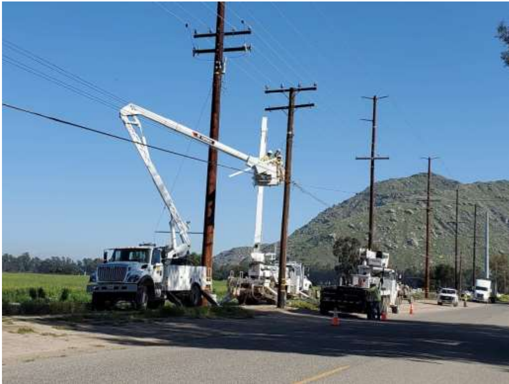
Photo 3 – Distribution cutover activities at Construction Area UNK25 (April 28, 2020).
