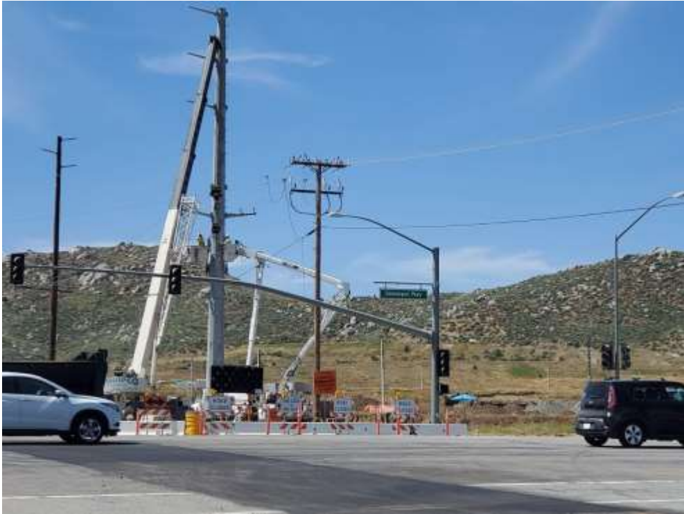
Photo 1 – Setting TSP at Construction Area UNK47 (May 6, 2020).
