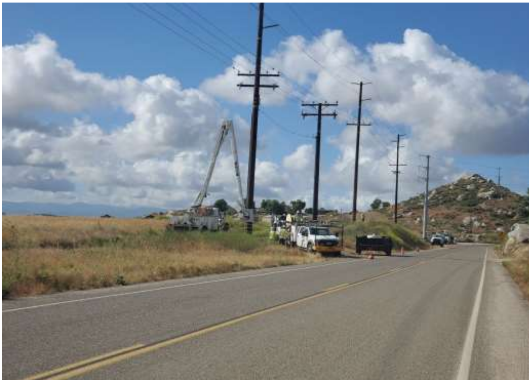
Photo 2 – Underground riser activities at Construction Area UNK112 (May 19, 2020).
