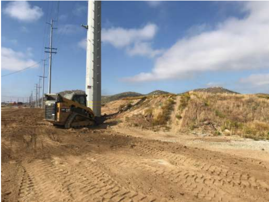
Photo 1 – Slope recontouring at Construction Area UNK41 (May 15, 2020) (Photo courtesy of SCE).
