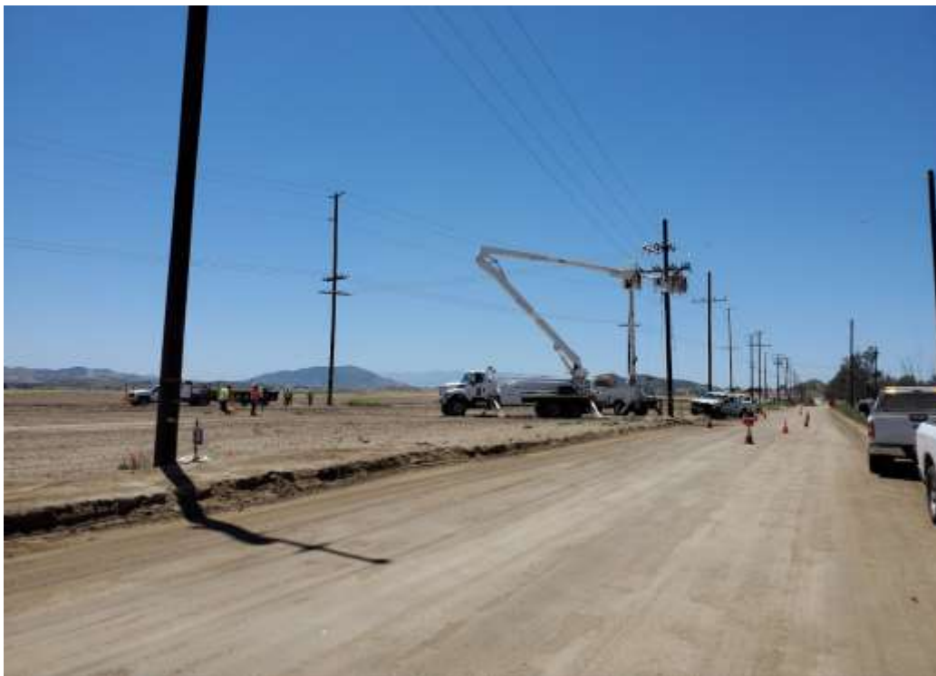
Photo 2 – Wire wreck-out activities at Construction Area UNK93 (May 26, 2020).
