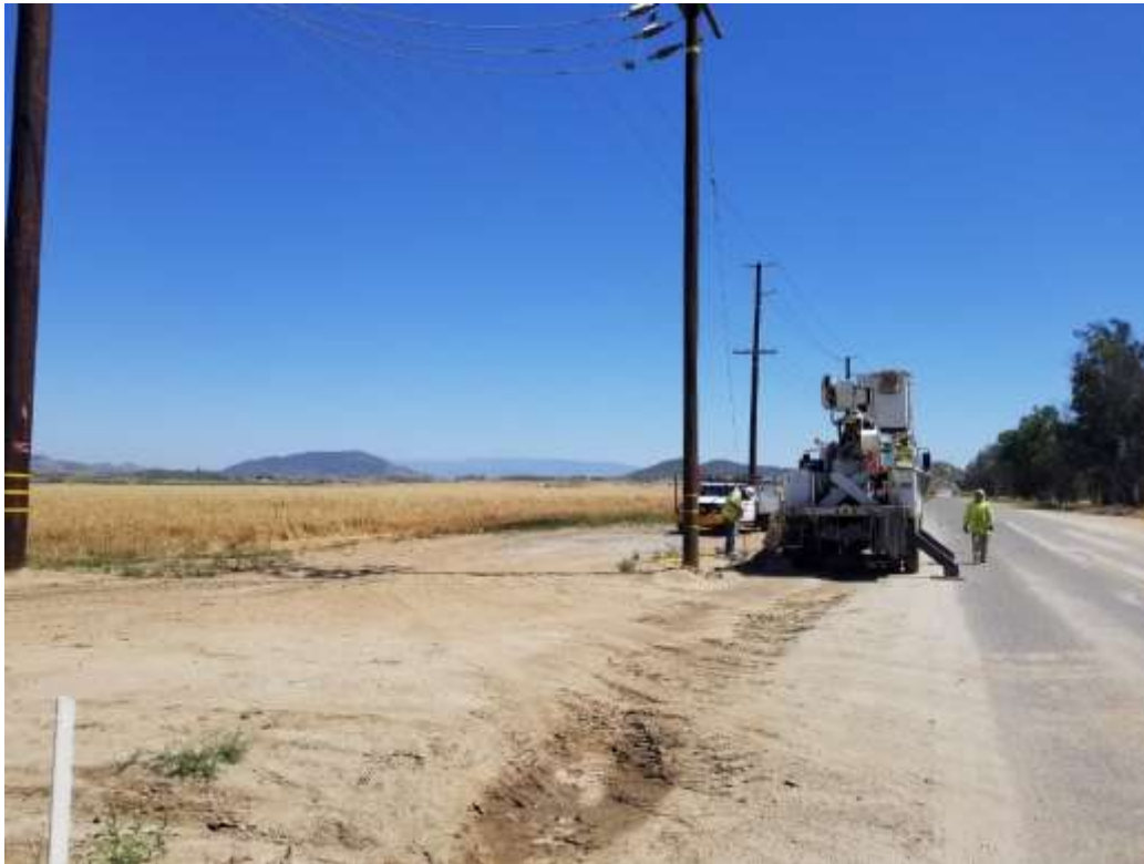
Photo 1 – Anchor replacement at Construction Area UNK98 (May 27, 2020) (Photo courtesy of SCE).
