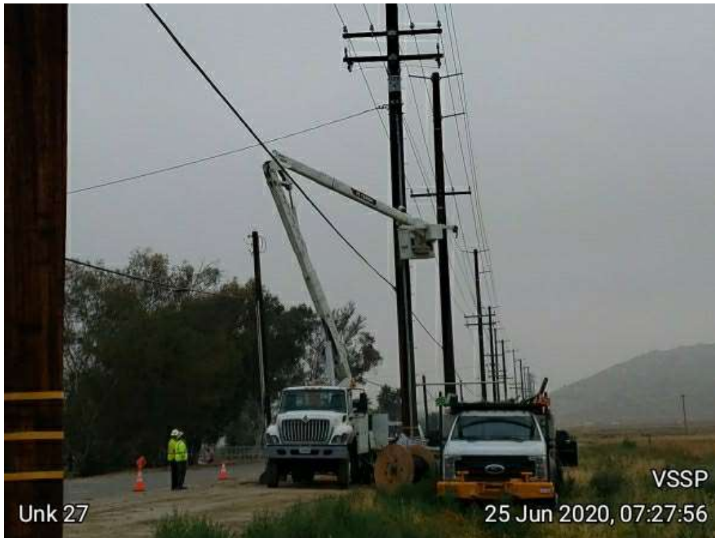
Photo 3 – Handhold installation at Construction Area UNK27 (June 25, 2020) (Photo courtesy of SCE).
