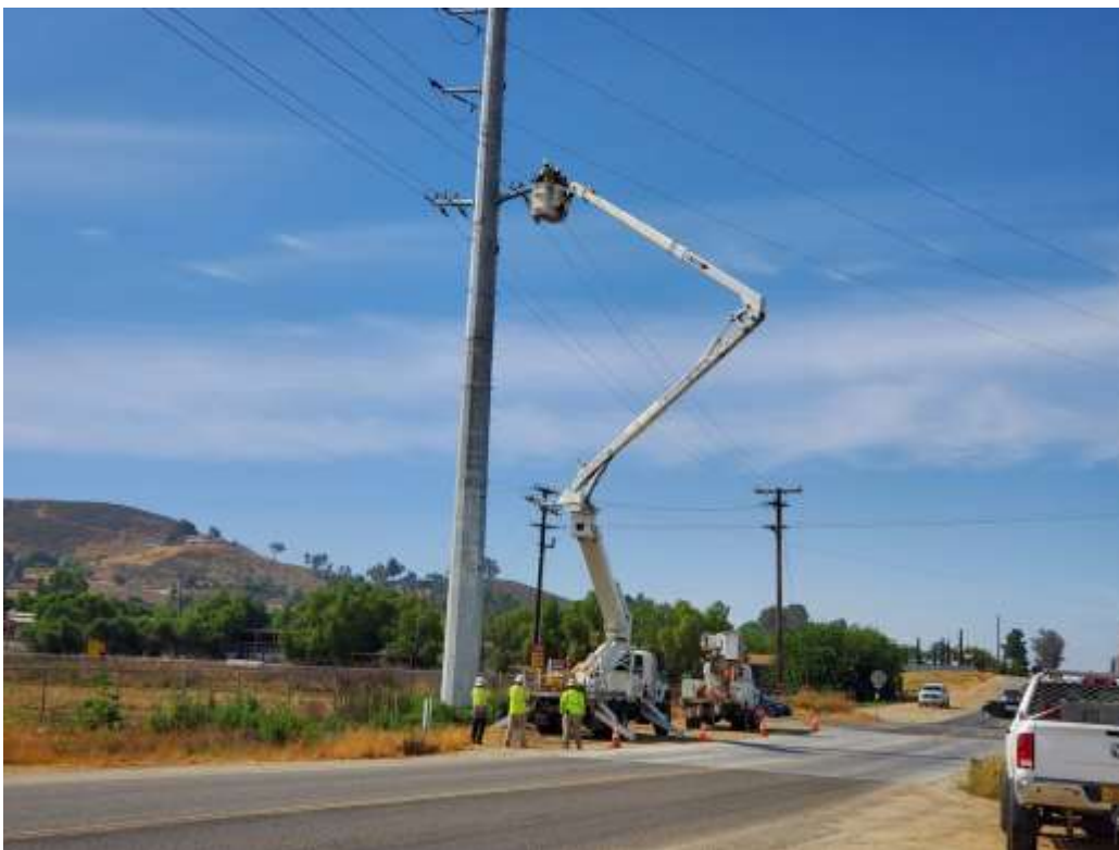
Photo 2 – Bird guard installation at Construction Area UNK154 (June 24, 2020).
