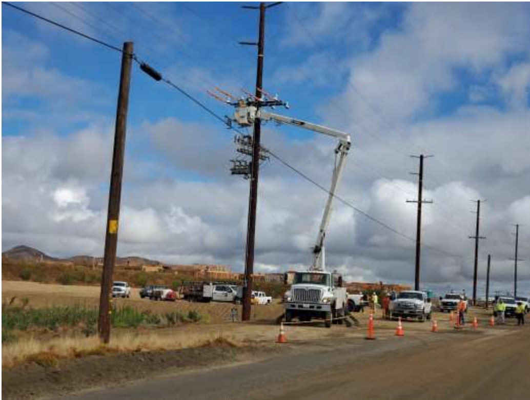
Photo 1 – RAR installation at Construction Area UNK56 (June 29, 2020).
