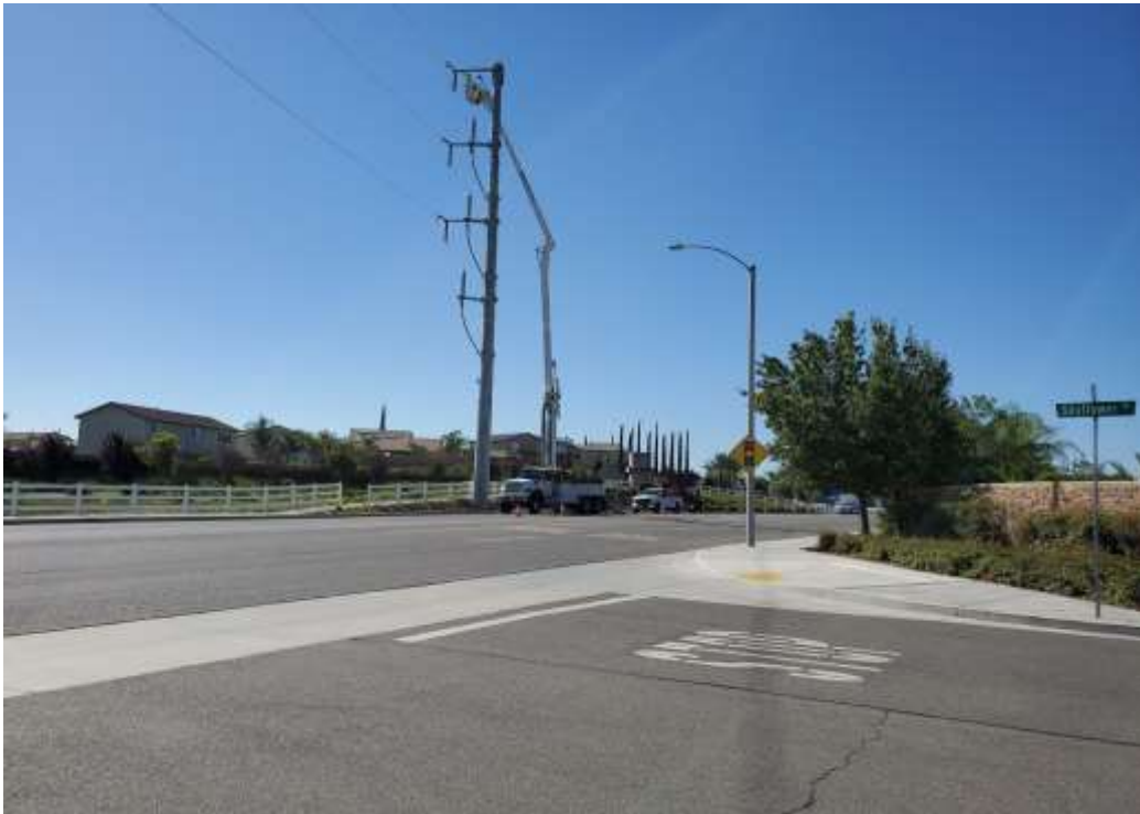
Photo 1 – Rolling phases at Construction Area UNK207 (August 10, 2020).
