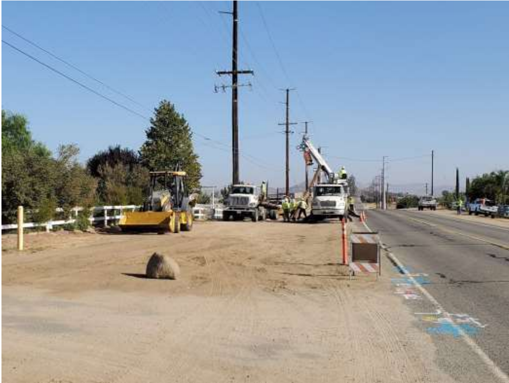
Photo 1 – Pole butt removal at Construction Area UNK159 (August 31, 2020).
