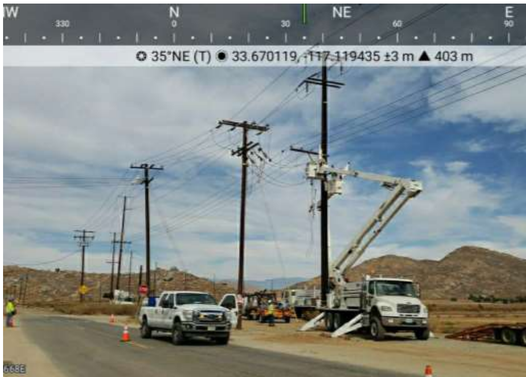
Photo 2 – Engineering fix at UNK98 (November 5, 2020) (Photo courtesy of SCE).
