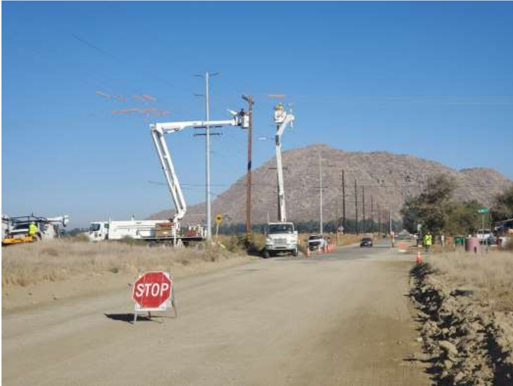
Photo 1 – Lowering distribution arms at Construction Area UNK35 (November 19, 2020).
