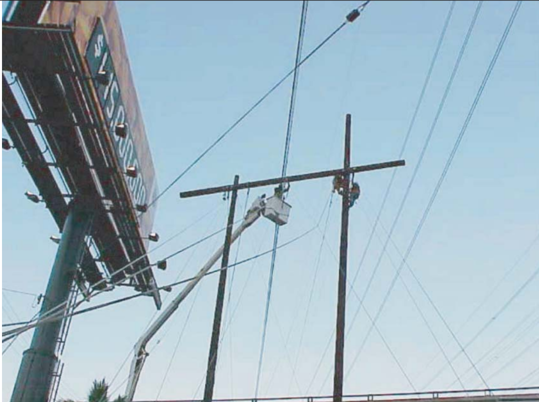
Low Voltage or Street Under-Crossing (H-Frame Configuration)
