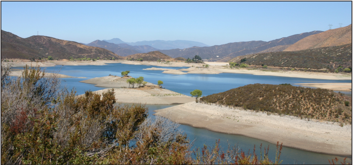
7 Existing transmission line corridor crossing dam (middle right) at Bouquet Reservoir.
