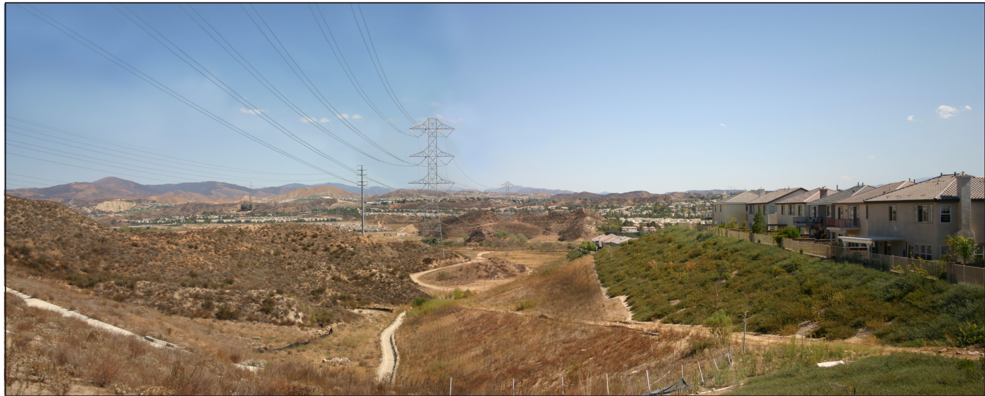
B 500 kV transmission line replacement as seen from KVA Seg 1-8.
