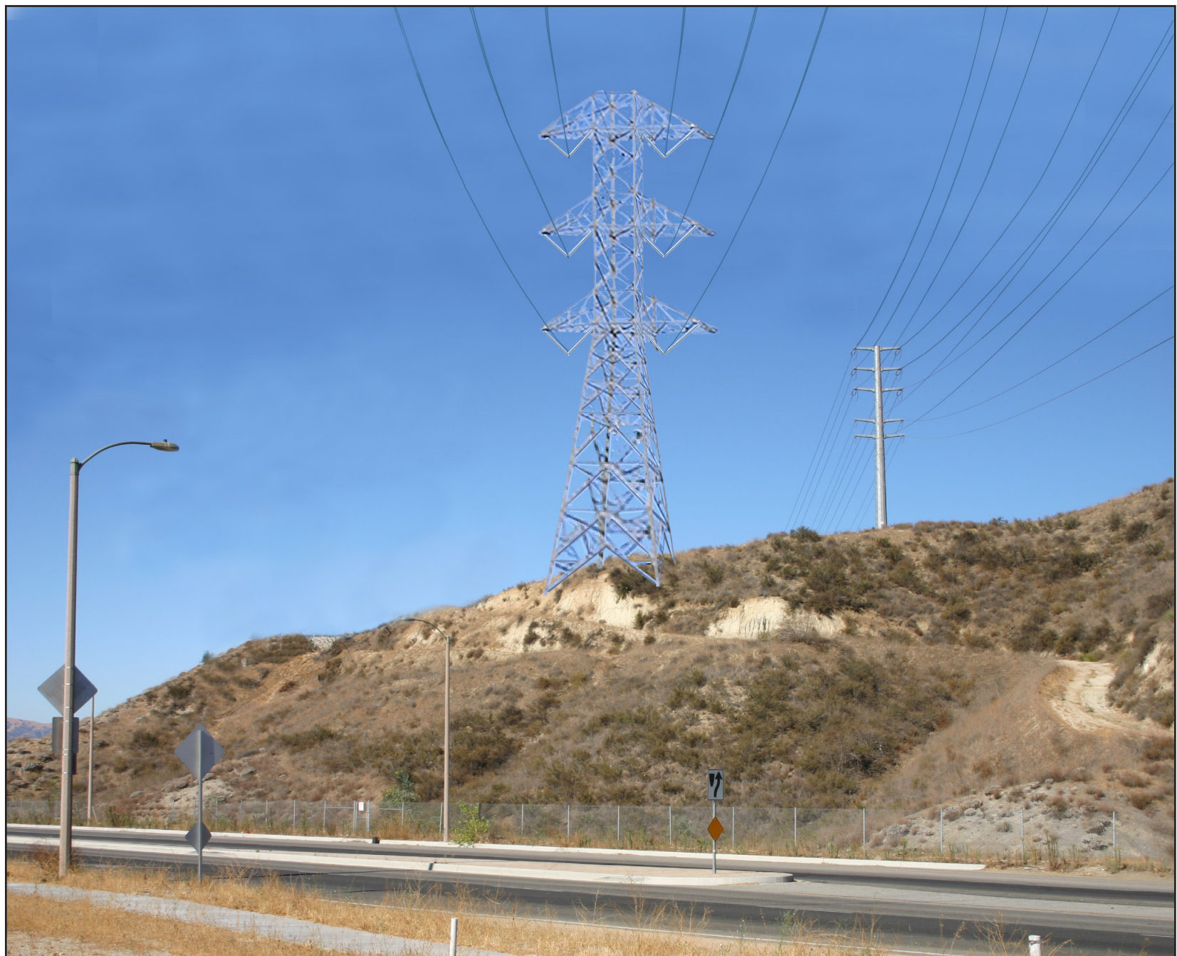
B 500 kV transmission line replacement as seen from KVA Seg 1-9.
