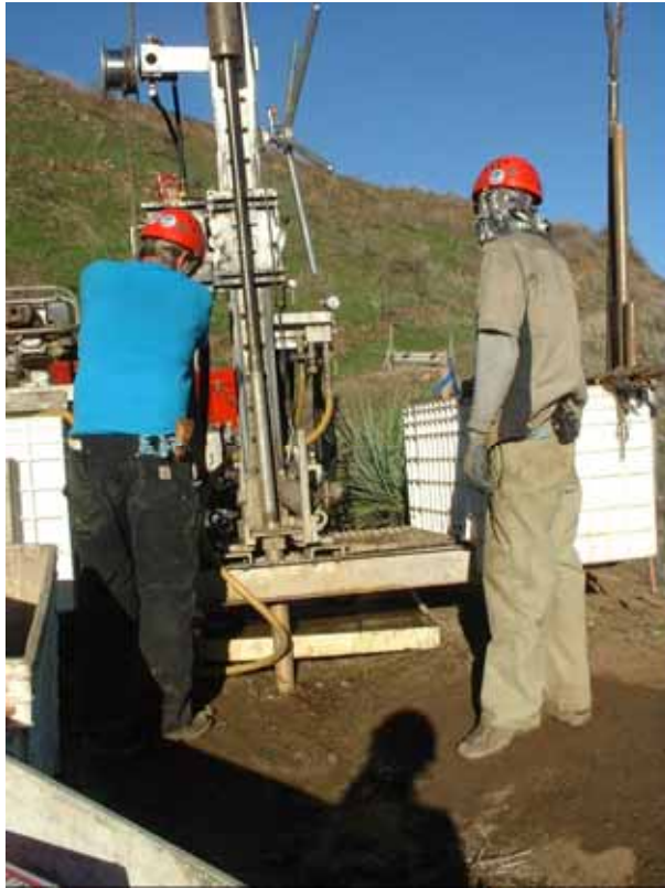
Figure 1: Drilling Operations at Tower Site 33.
