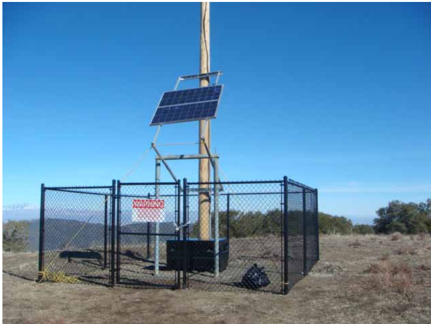
Figure 2: Radio Repeater Tower after damage repaired due to high winds.
