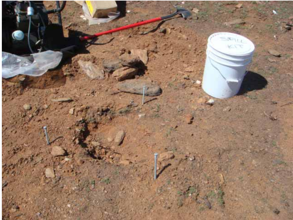
Figure 1: Removal of gasoline spill and contaminated soils at Tower Site 50.
