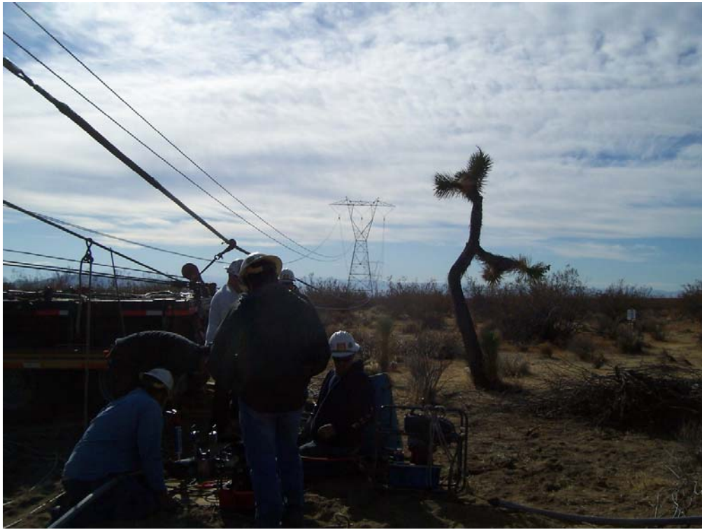
Figure 3: Segment 3 wire stringing and sleeving activities between Towers 16-26.
