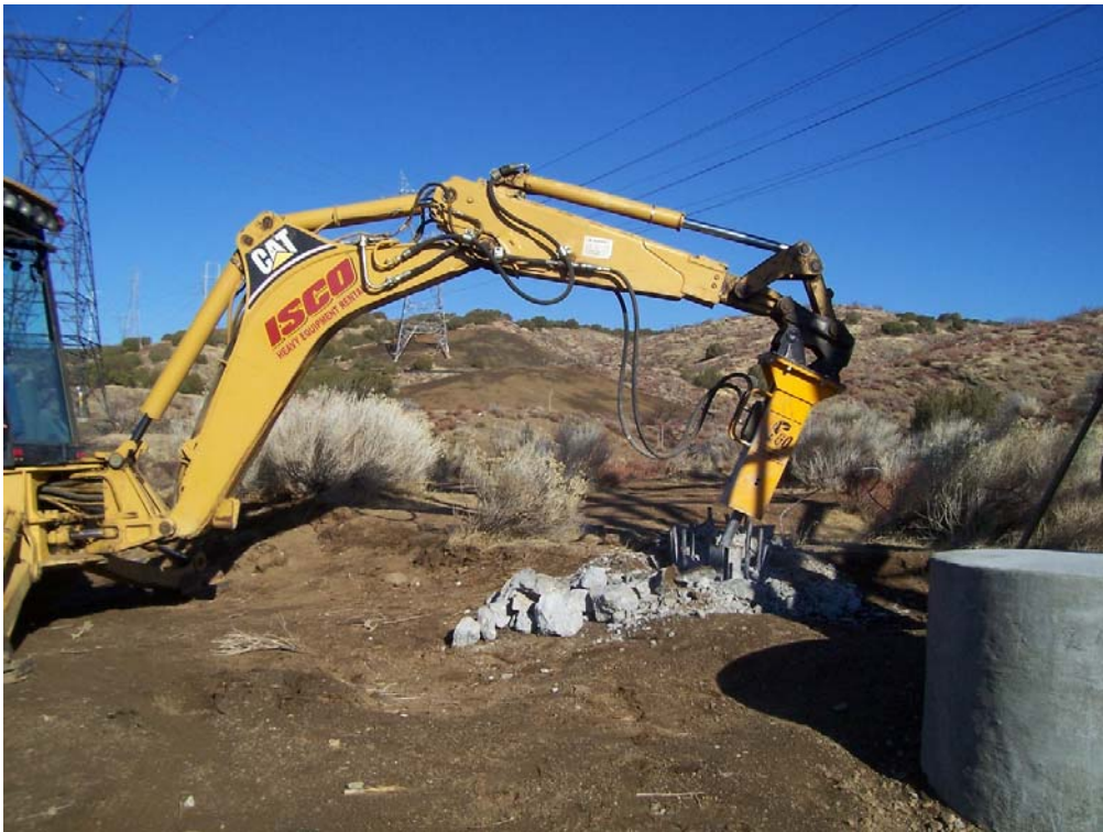
Figure 2: Wreck-out tower footer removal near Tower 34A, Segment 2.
