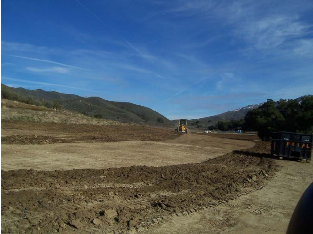
Figure 1: Hydrant yard soil decompaction in preparation for revegetation, Segment 1..
