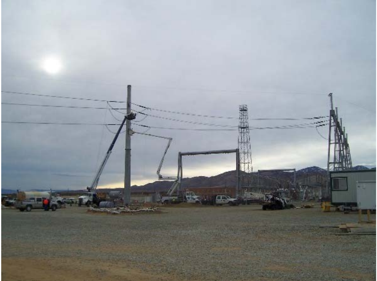
Figure 4: Wire stringing inside Windhub Substation on the temporary Bypass structures.
