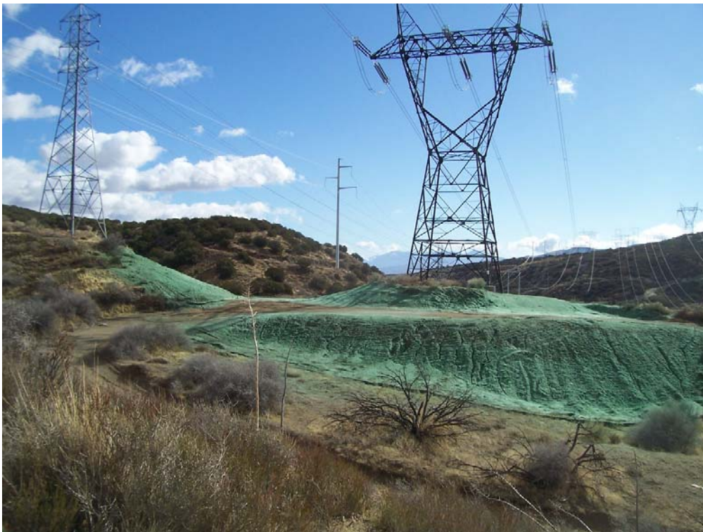
Figure 2: Hydroseed application for erosion control at Tower 34A, Segment 2.
