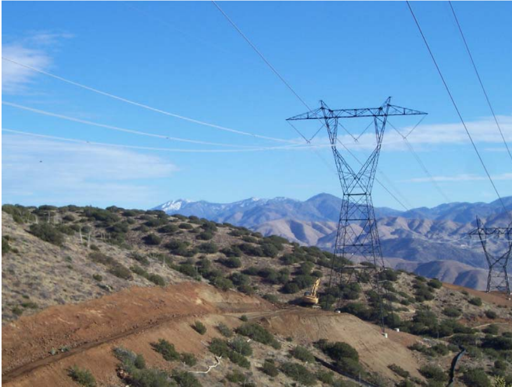
Figure 1: Recontouring at Tower 95, Segment 2.
