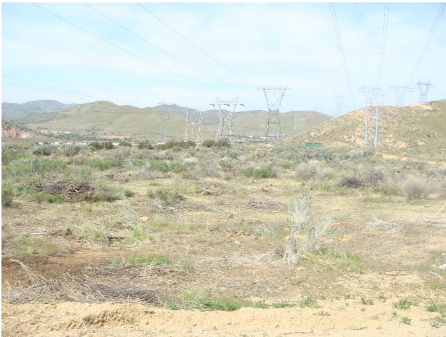
Figure 2: Vegetation clearing at the Vincent Substation expansion area. Further vegetation removal is on hold pending CDFG concurrence of a reduced buffer for nesting birds or until birds have fledged.
