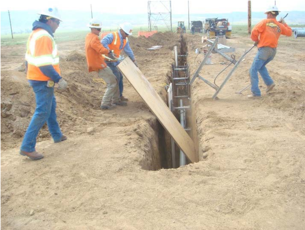
Figure 1: Underground relocation of the 66 kV line outside of the Antelope Substation.
