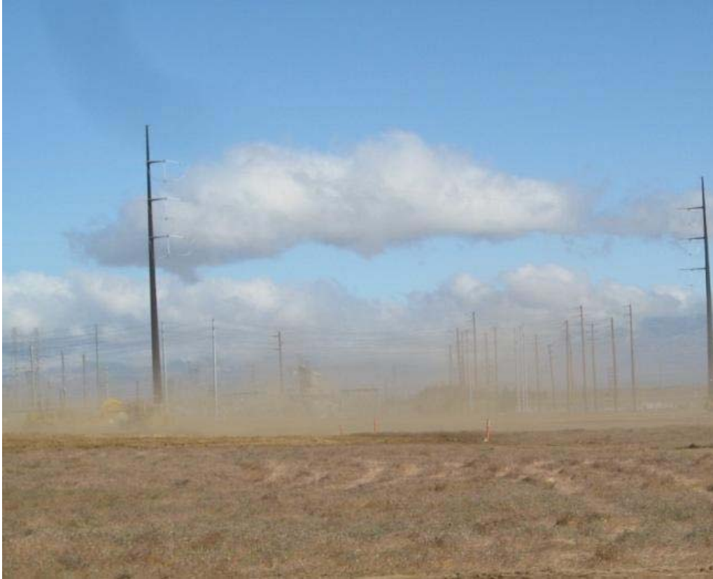
Figure 1: Fugitive dust observed during grading activities at the Antelope substation expansion area.
