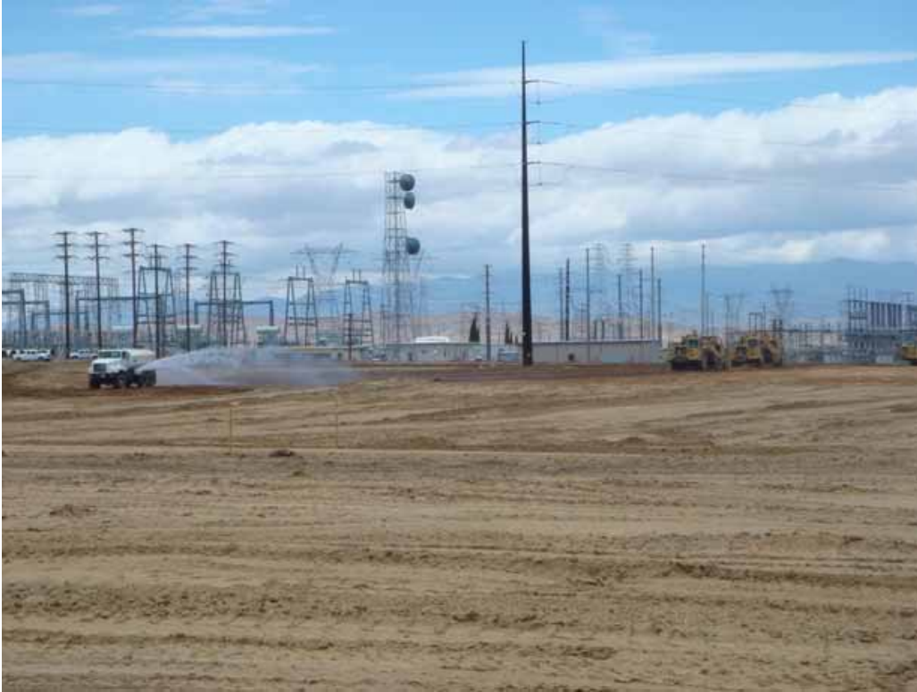
Figure 1: Continued construction at the Antelope Substation expansion area.
