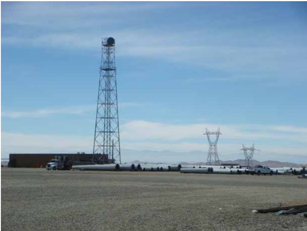
Figure 2: Materials stored at the Windhub Substation adjacent to the microwave tower and MEER building.
