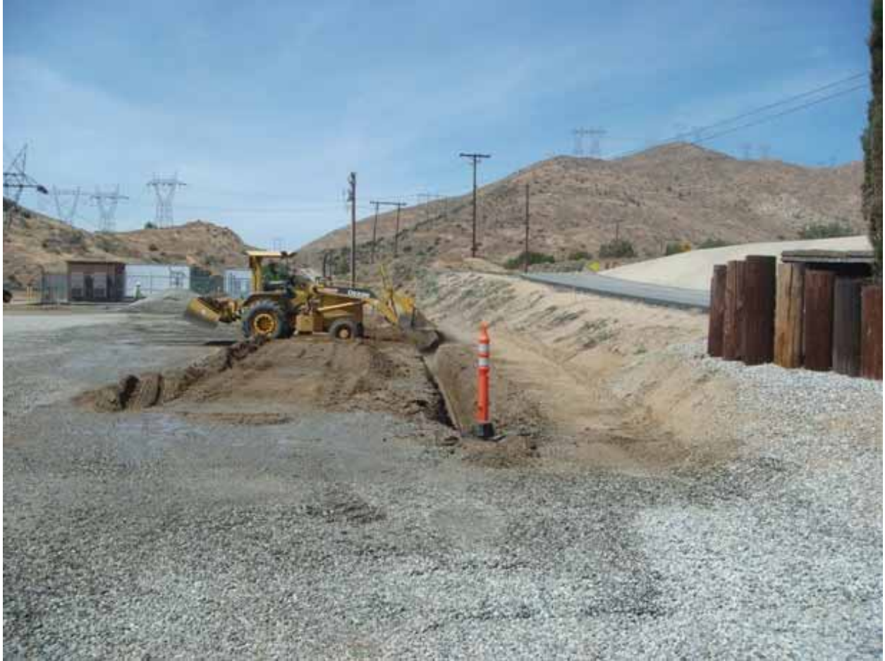
Figure 3: Trenching work taking place at the Vincent Substation.
