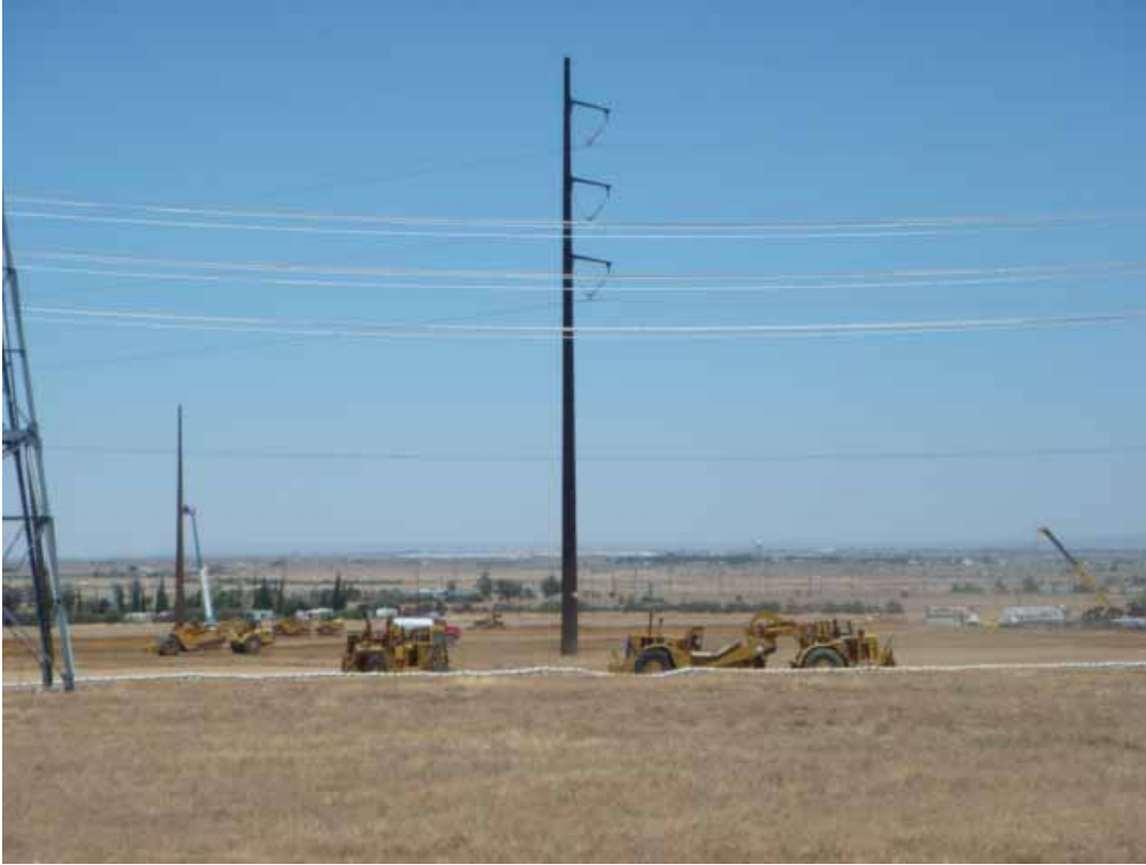
Figure 1: Grading continued at the Antelope Substation.
