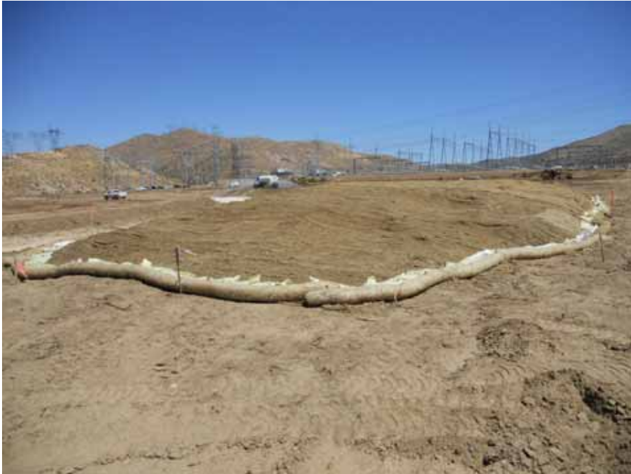
Figure 1: Topsoil pile at Vincent Expansion.
