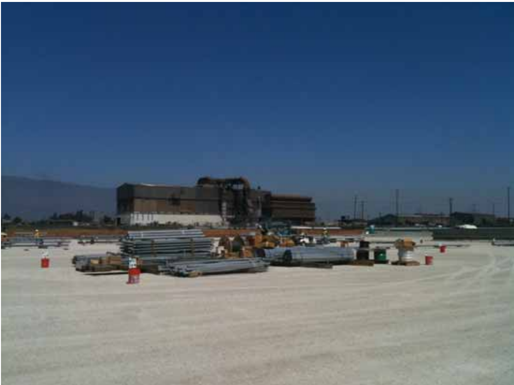
Figure 2: Material storage in Rancho Vista Yard.
