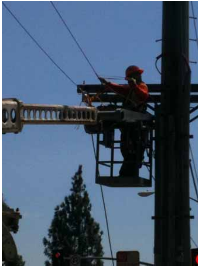
Figure 4: Segment 8 Telecom aerial work along in Pomona.
