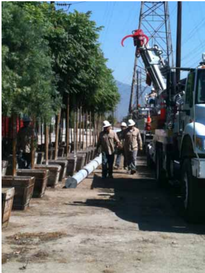
Figure 5: Segments 7/8 66 kV poles placed along the right-of-way.
