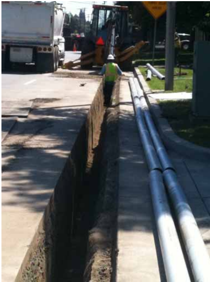
Figure 3: Segment 8 Telecom trenching work along Peyton Drive in Chino Hills.
