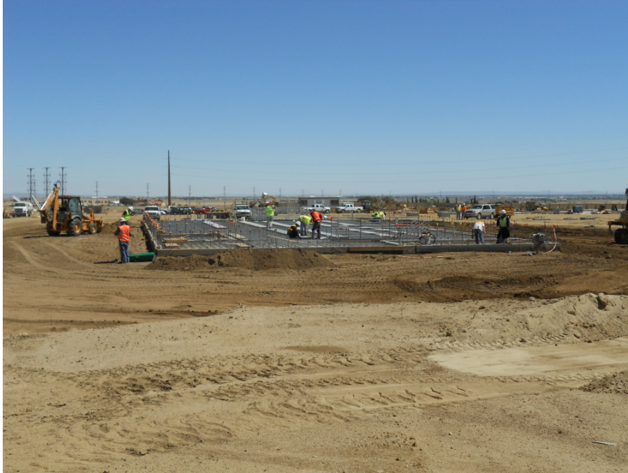
Figure 1: Construction of the MEER building in the Antelope Substation Expansion, Segment 1.
