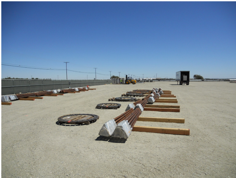
Figure 2: Material storage at Material Yard 28 on Avenue I.
