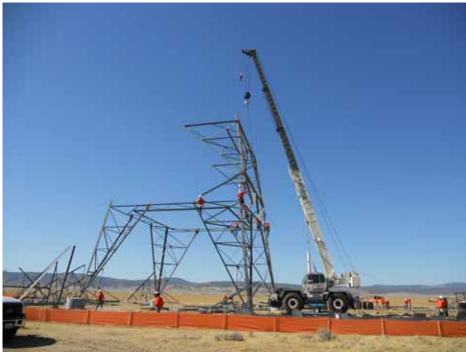
Figure 2: Segment 4, Tower 34 assembly.
