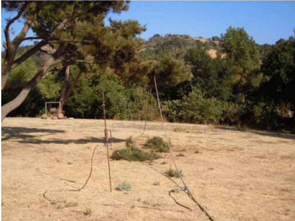
Figure 4: Unintentional 220 kV (de-energized) wire drop in Tonner Canyon.
