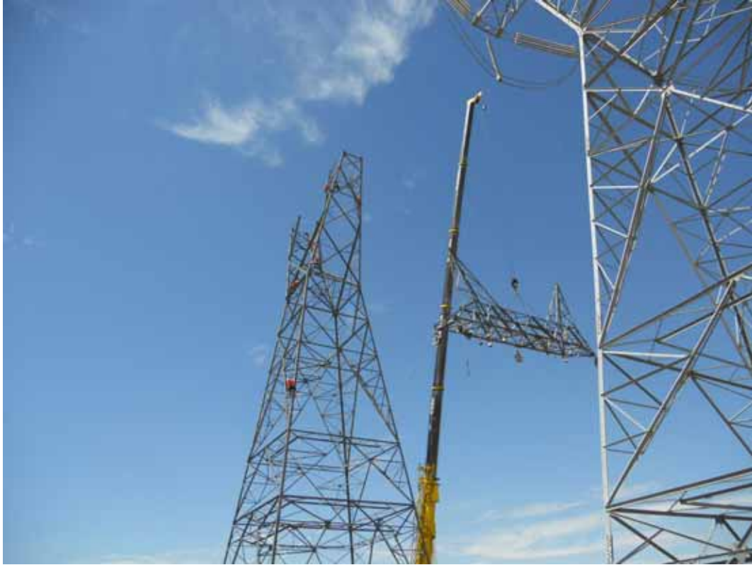
Figure 1: Segment 4, Tower 34 bridge installation
