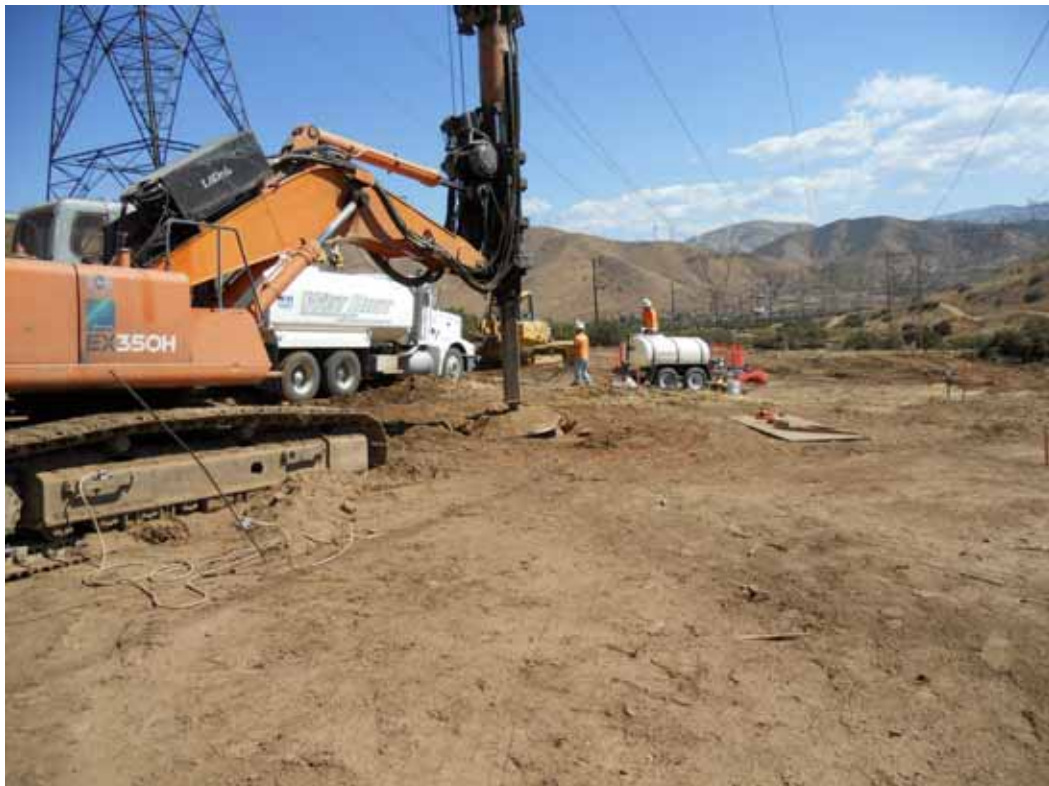
Figure 2: Segment 5, Tower 61 foundation drilling
