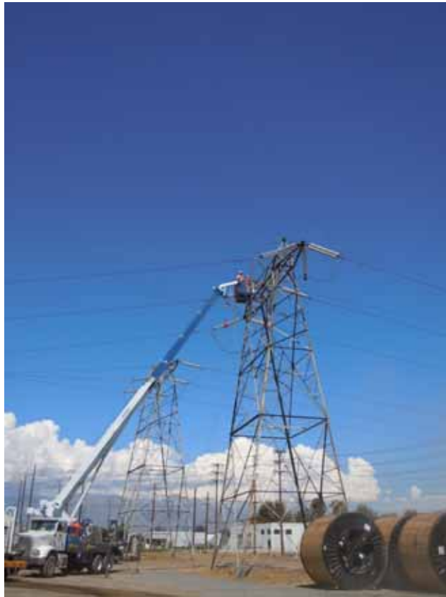
Figure 5: Segment 8 Phase 2, crews remove hardware at M0-T2 adjacent to Chino Substation.
