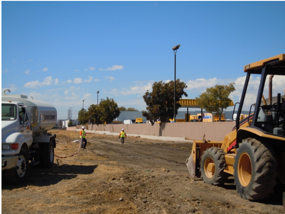
Figure 6: DCX crews prepare the Chino Yard for contractor equipment storage.
