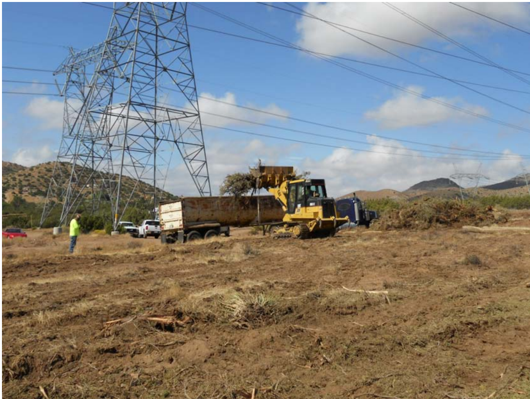
Figure 2: Segment 5, juniper stockpile removal near Tower 61.
