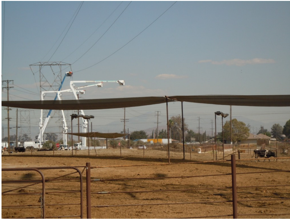
Figure 5: Crews remove hardware at M3-T3 adjacent to a dairy, Segment 8 Phase 2.
