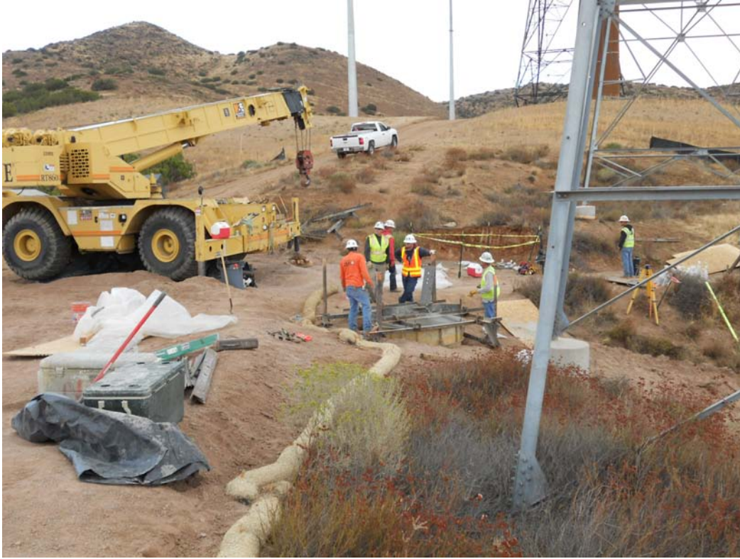
Figure 1: Segment 5, Tower 60 concrete form at new tower foundation.
