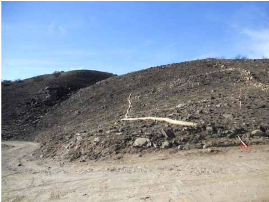
Figure 2: Segment 5: BMP (fiber roll) installation at Tower 31.
