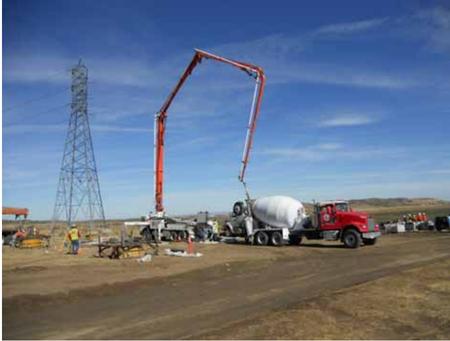
Figure 3: Woodward crew pouring concrete in foundations at Tower 39, Segment 5.
