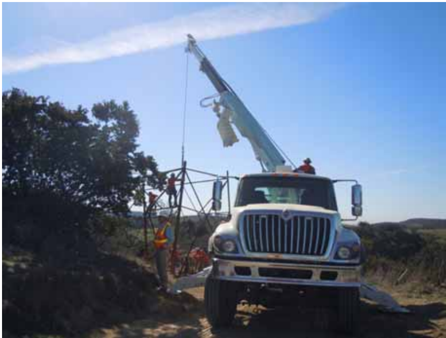
Figure 5: A Wilson crew dismantles Tower M58-T1 in Tonner Canyon, Segment 8, Phase 1.
