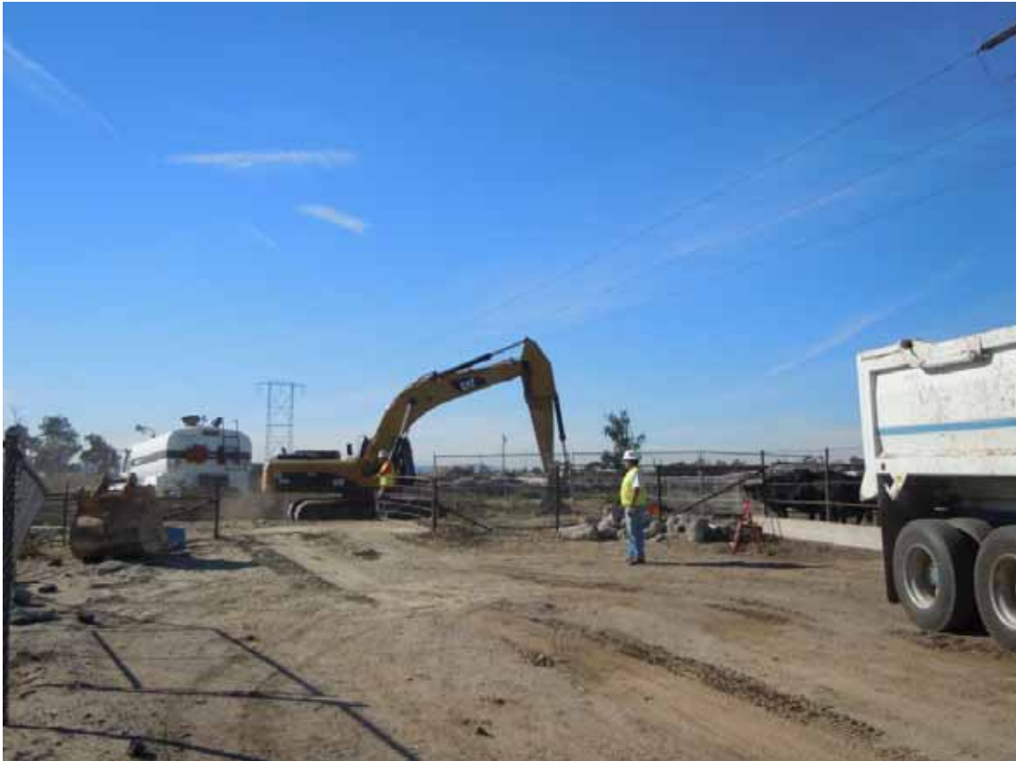
Figure 5: A DCX crew removes a footer at Tower M3-T4, Segment 8 Phase 2.
