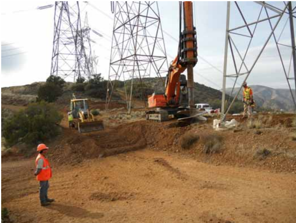
Figure 2: Woodward (drilling subcontractor) drilling foundations at Tower 54 on Segment 5.
