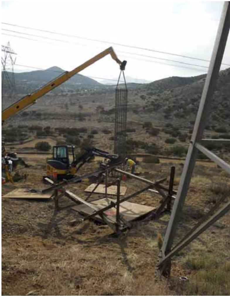
Figure 3: Woodward setting rebar cage at Tower 59 on Segment 5.
