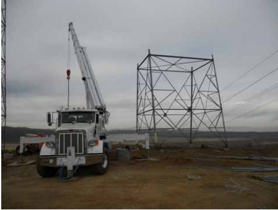
Figure 1: Wrecking out existing 220 kV tower, M69-T3, Segment 5.
