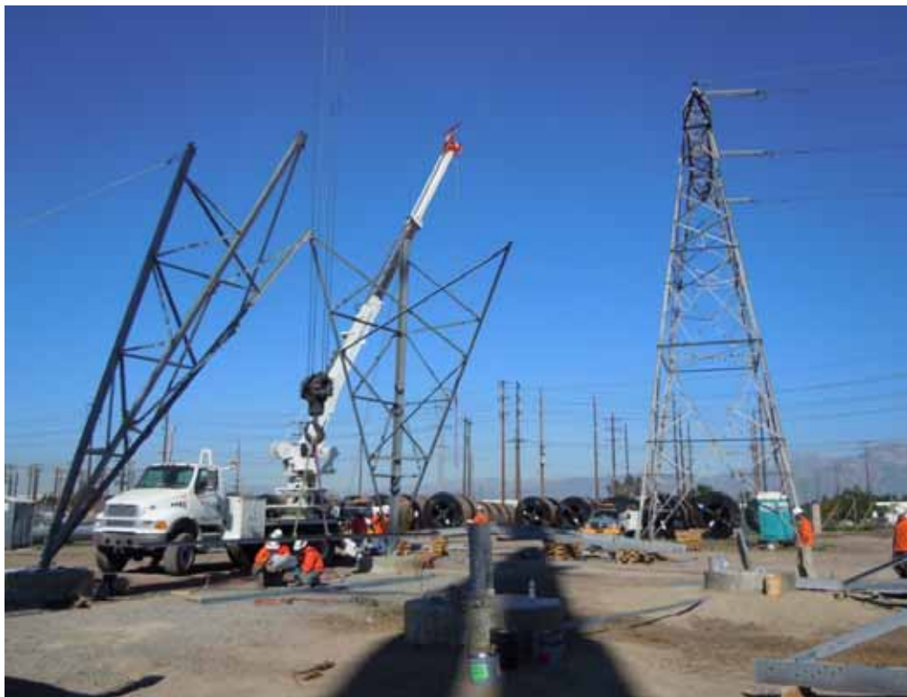
Figure 6: A Wilson crew assembles new tower at M0-T2, Segment 8, Phase 2.
