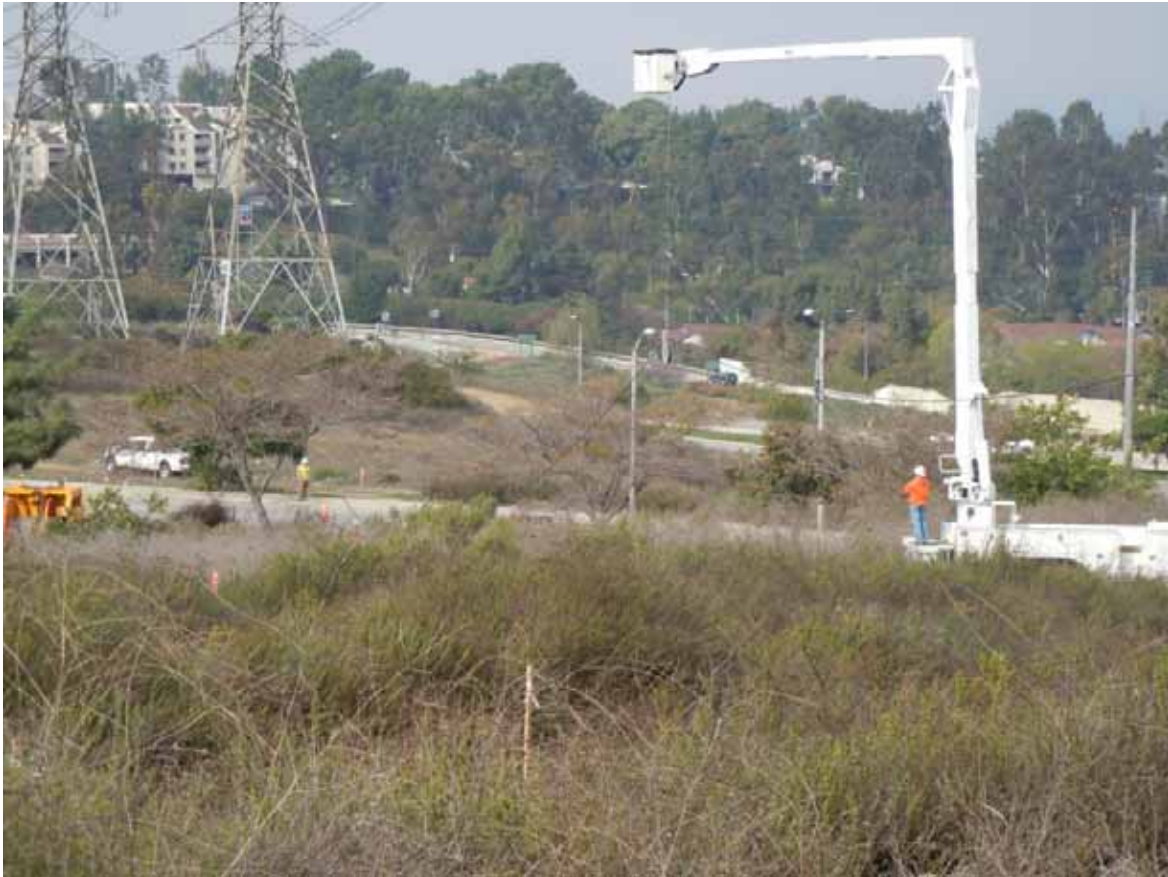
Figure 5: To avoid impacts to critical habitat for coastal California gnatcatcher, conductor was lowered into a traveler, Segment 7.
