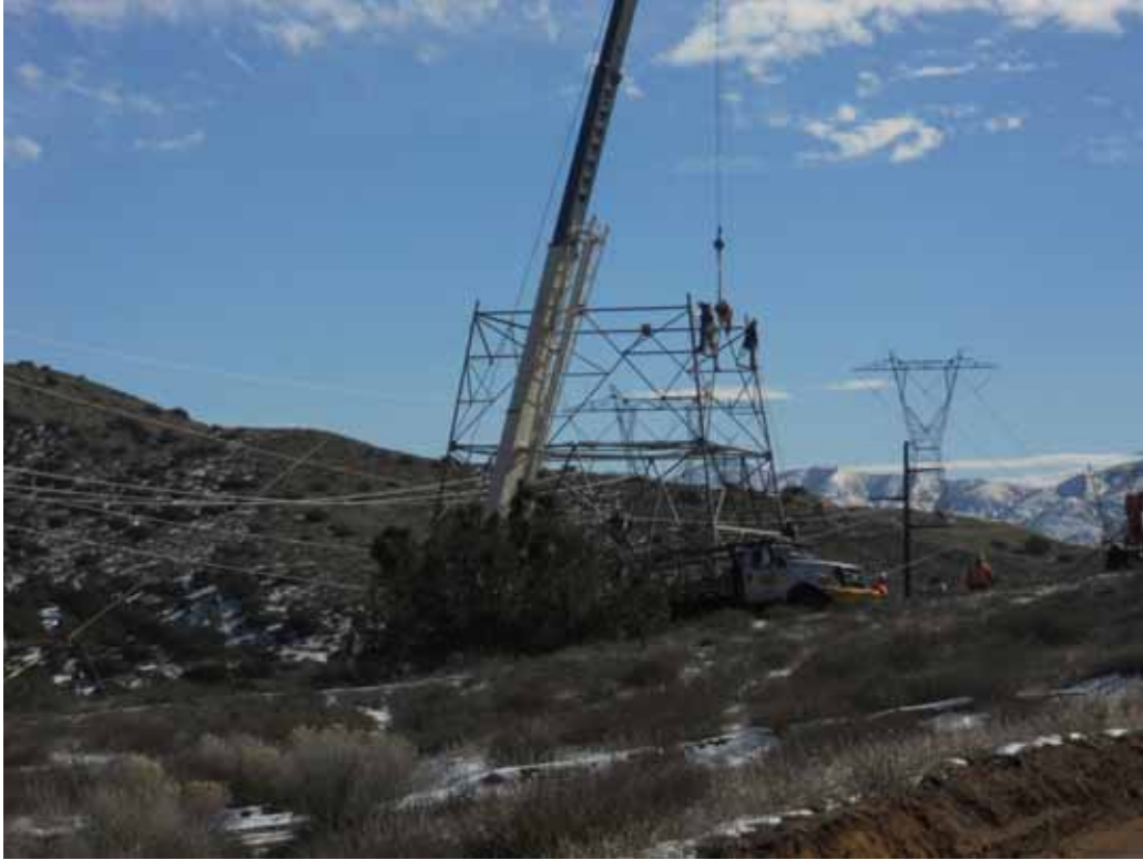
Figure 1: Assembly of 500 kV Tower 58, Segment 5.
