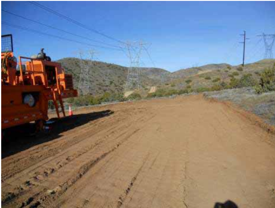
Figure 2: Graded wire pull site north of Tower 60, Segment 5.
