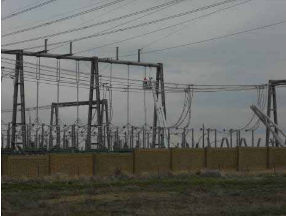
Figure 1: H&M wire crew preparing to remove conductor from Tower M59-T2A into a rack inside the Antelope Substation, Segment 5.
