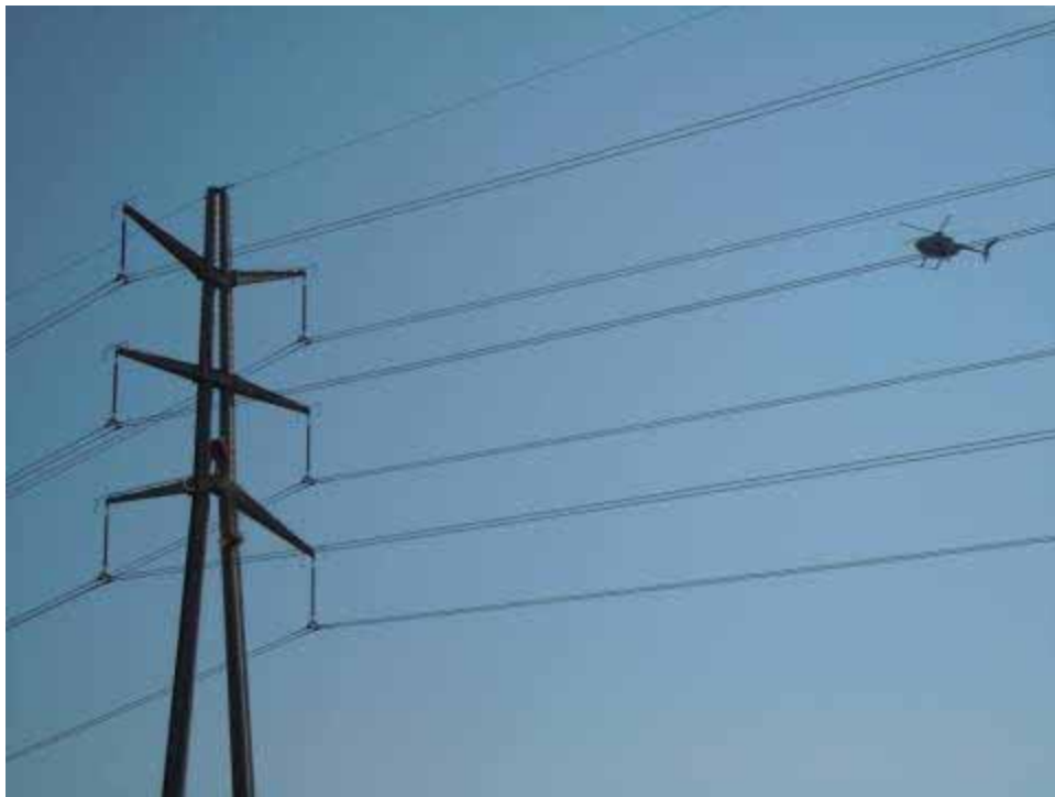
Figure 8: A Wilson lineman removes an inactive bird nest, Segment 8 Phase 3.
