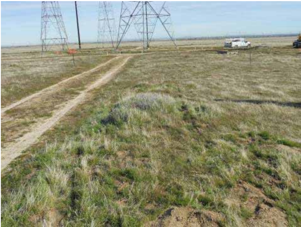
Figure 3: Tire tracks outside the approved disturbance limits at Tower 38, Segment 4.
